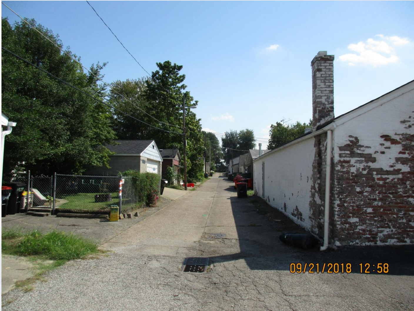
Alley to South
