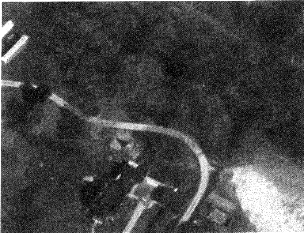
Figure 13. 2002 aerial image showing the footprint of the recently demolished cabin.
