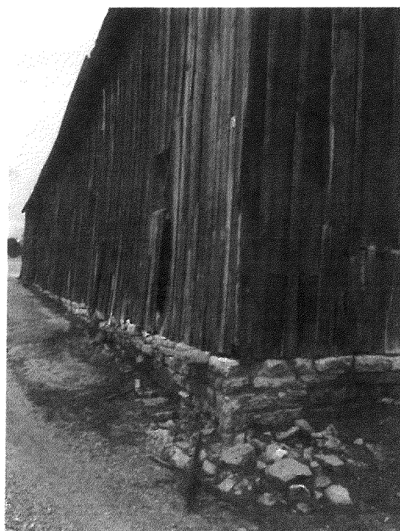
Figure 9. Barn with stone foundation.
