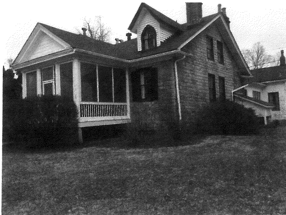
Figure 1. Yager House from front.
