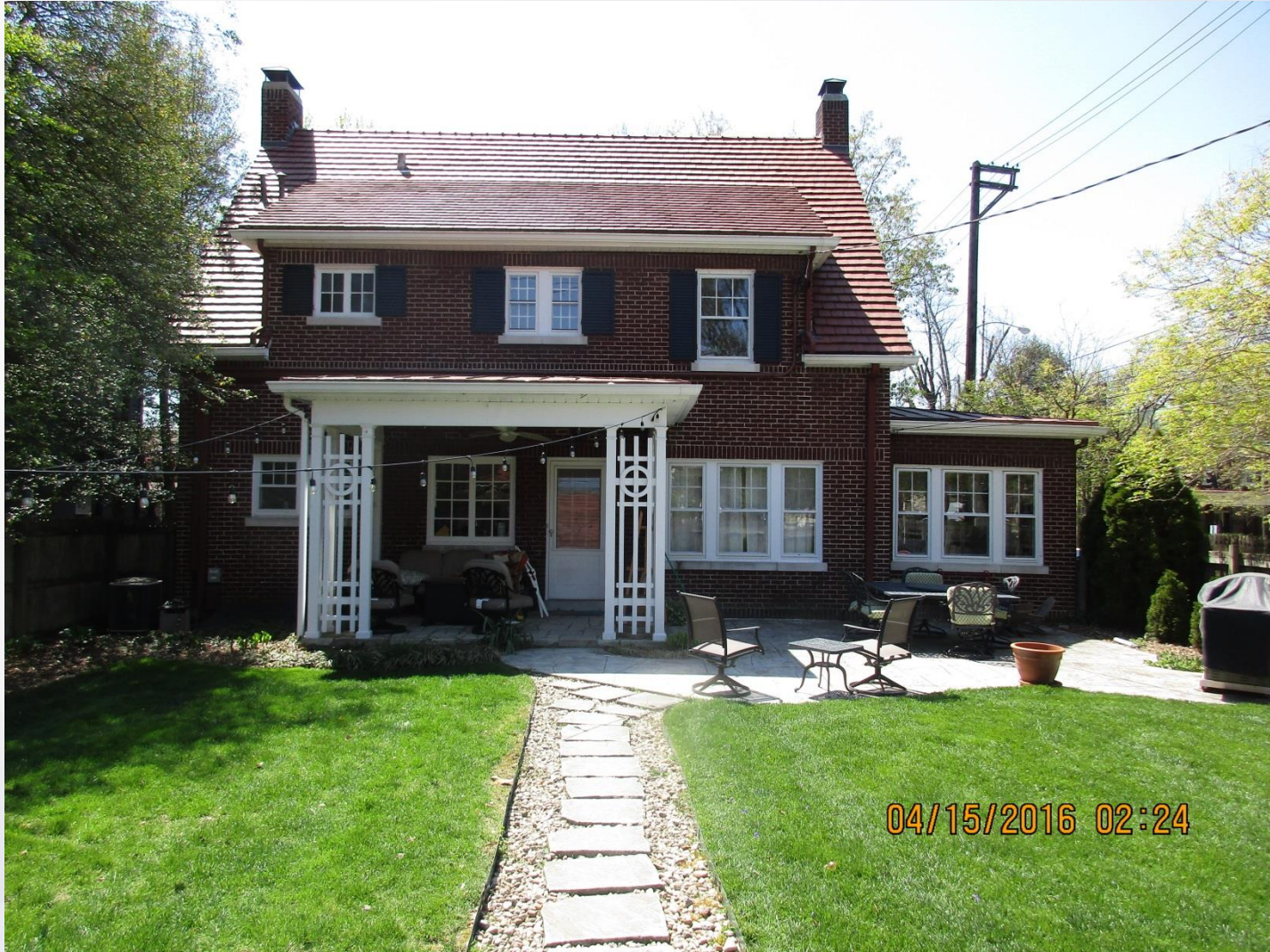
Looking at the rear of the principal structure where the proposed addition would be added.
