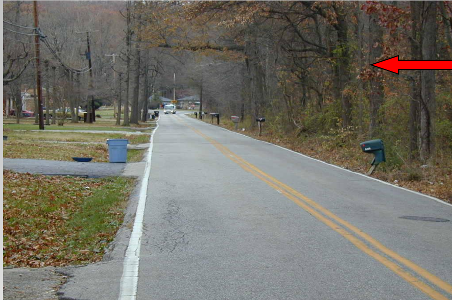
View Along McNair Road Looking West
