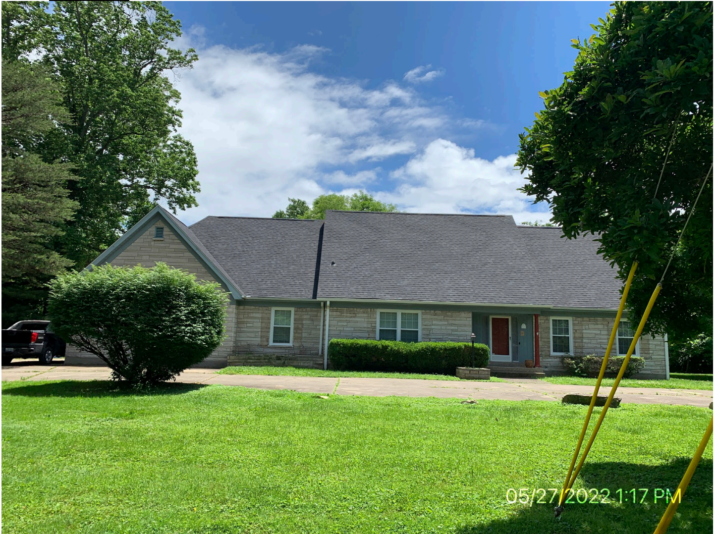
Front of subject property.
