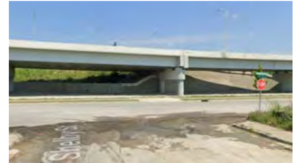
North Shelby Street facing north towards Witherspoon Street (Google Earth)
