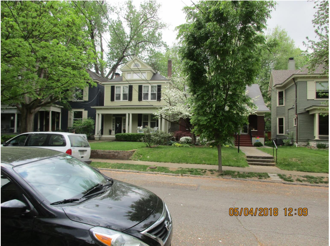
The properties across Bassett Avenue.
