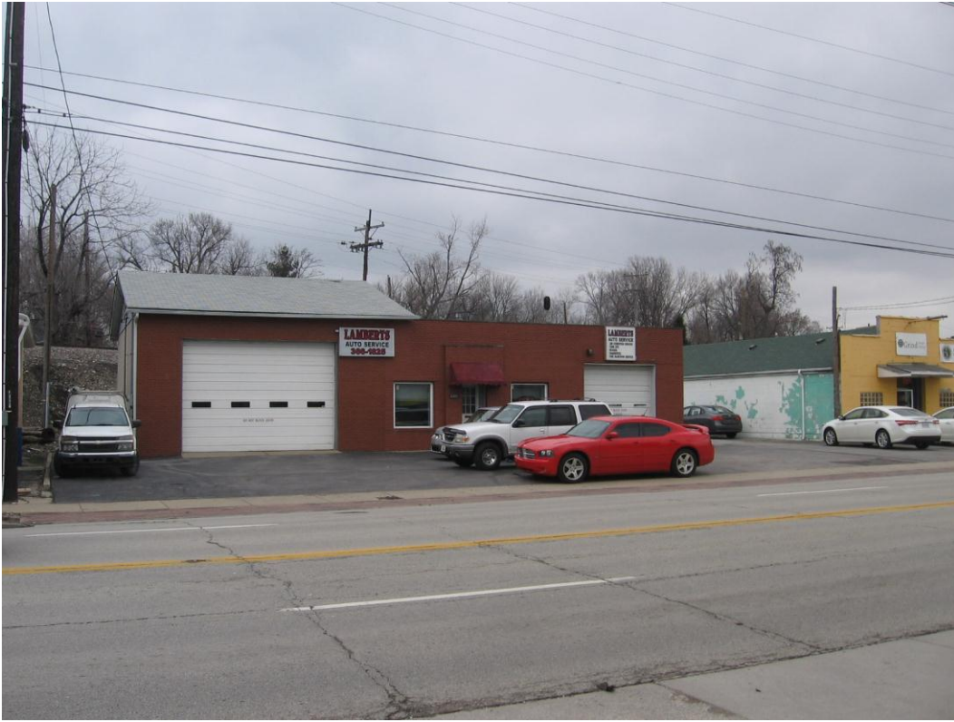
Existing businesses (looking east) across the street (Preston Highway) from the subject site
