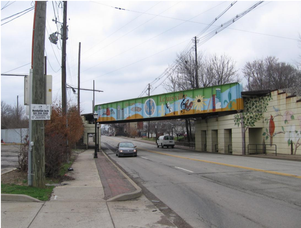
Looking north along Preston Highway frontage/ Existing street scape, plantings, and moral/ Location of proposed improved bus stop
