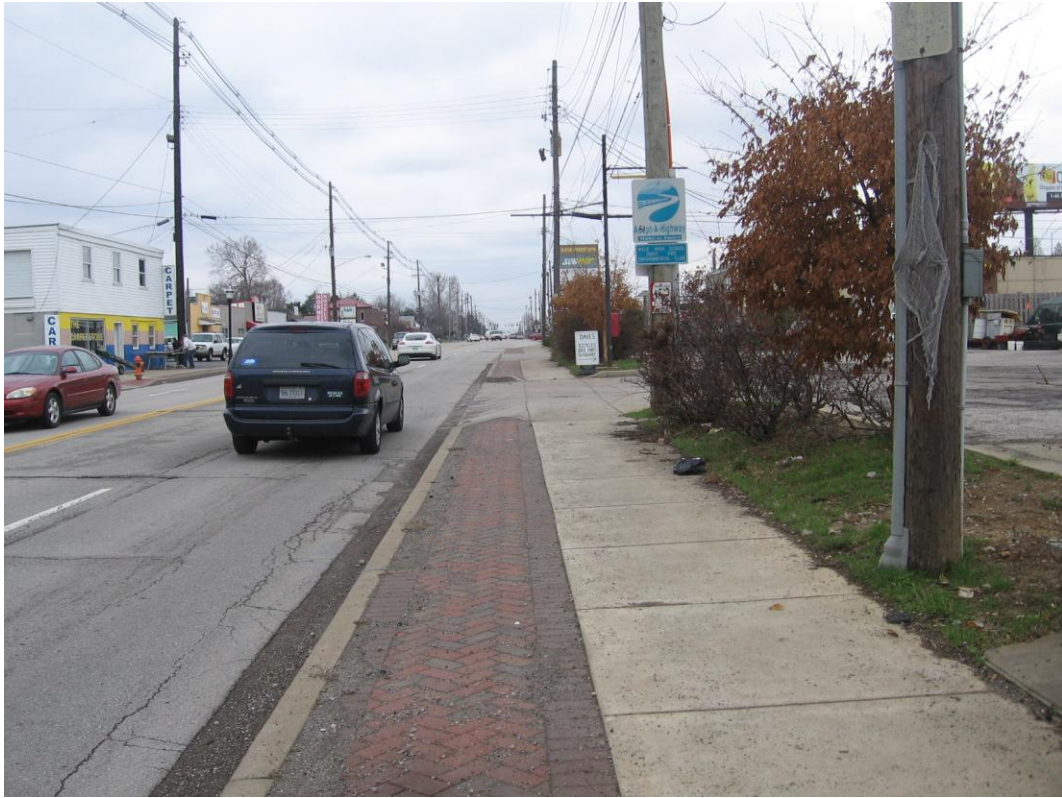
Looking south along Preston Highway frontage/ Existing street scape and plantings/ Location of proposed improved bus stop
