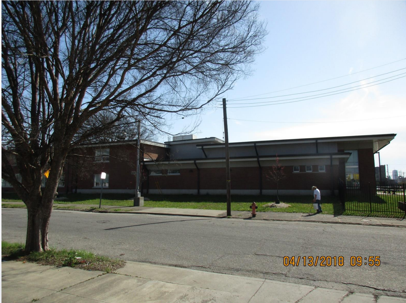
Looking east from the subject site towards the Elementary School, Roosevelt Perry Elem.
