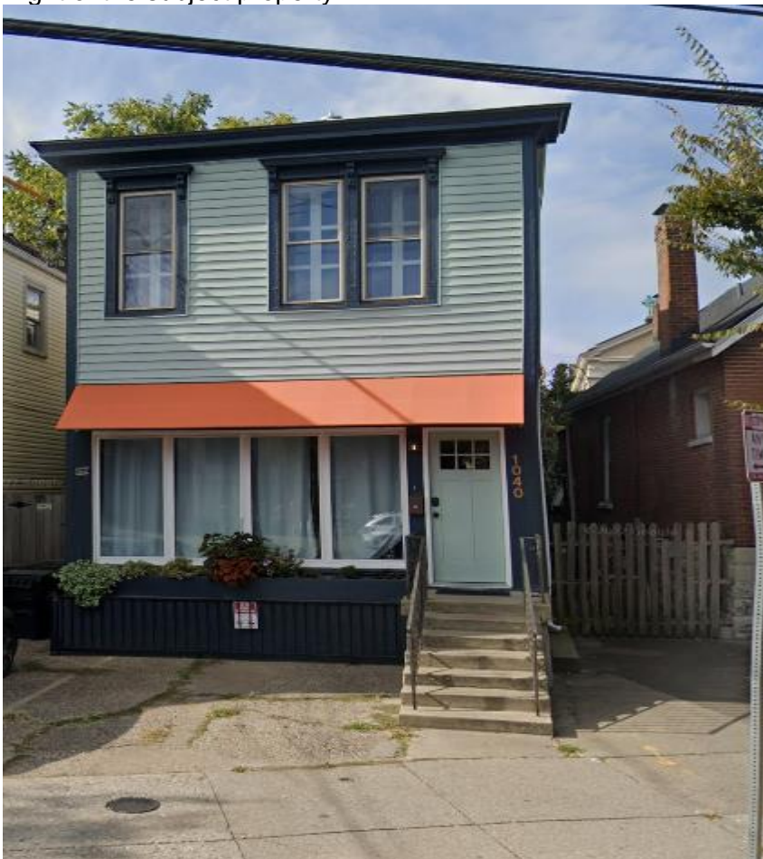
Left of subject property.
