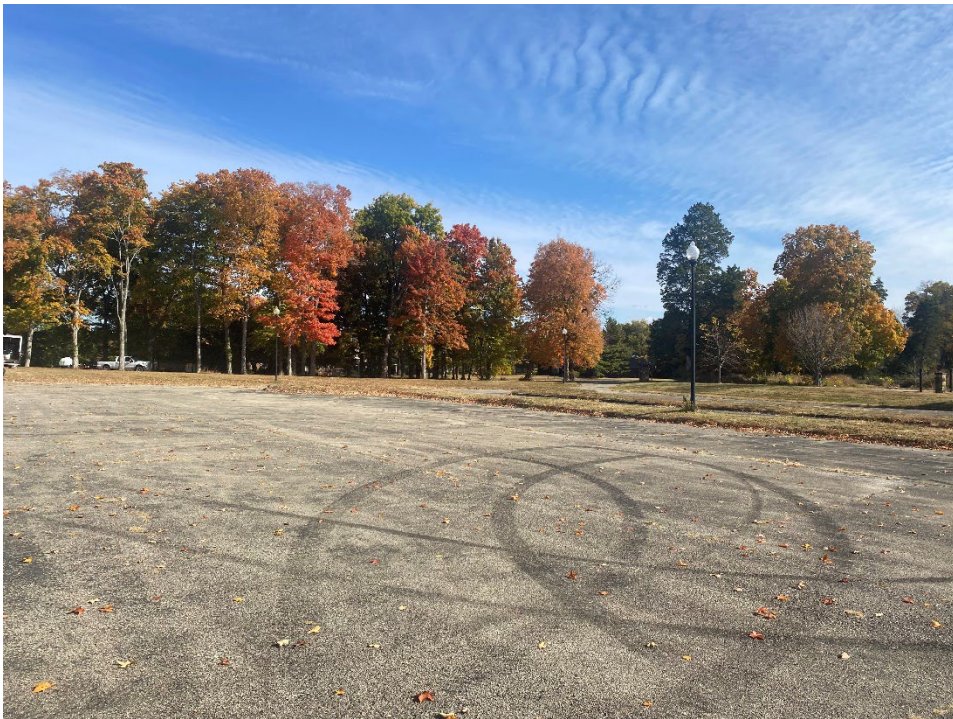
Existing parking lot
