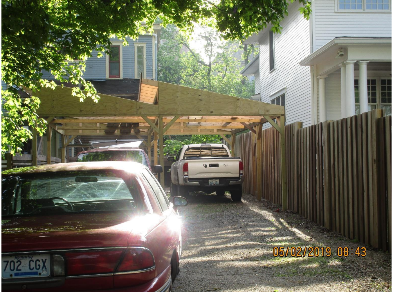
Variance area looking toward Peterson Avenue.
