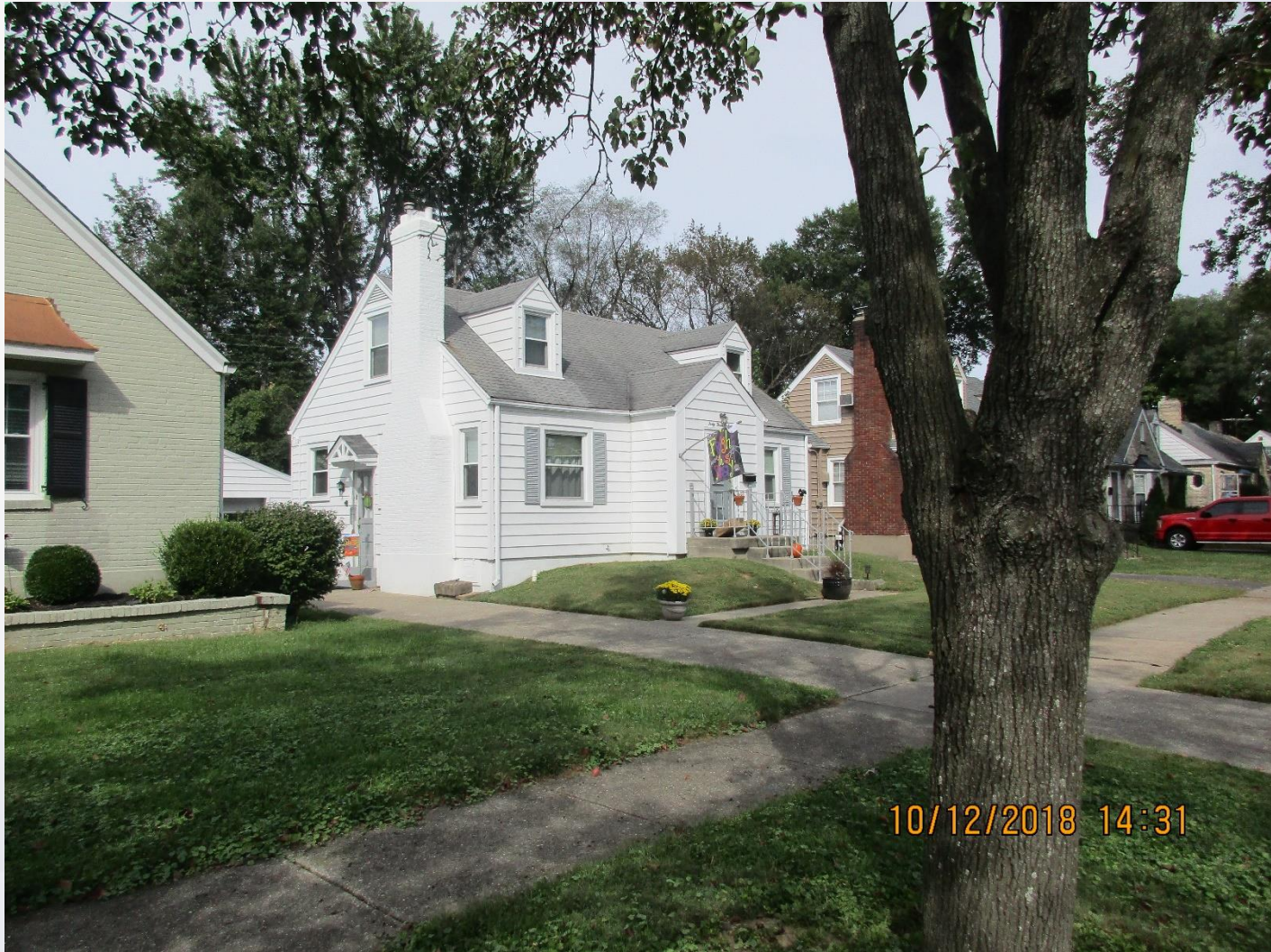
Adjoining Property to East
