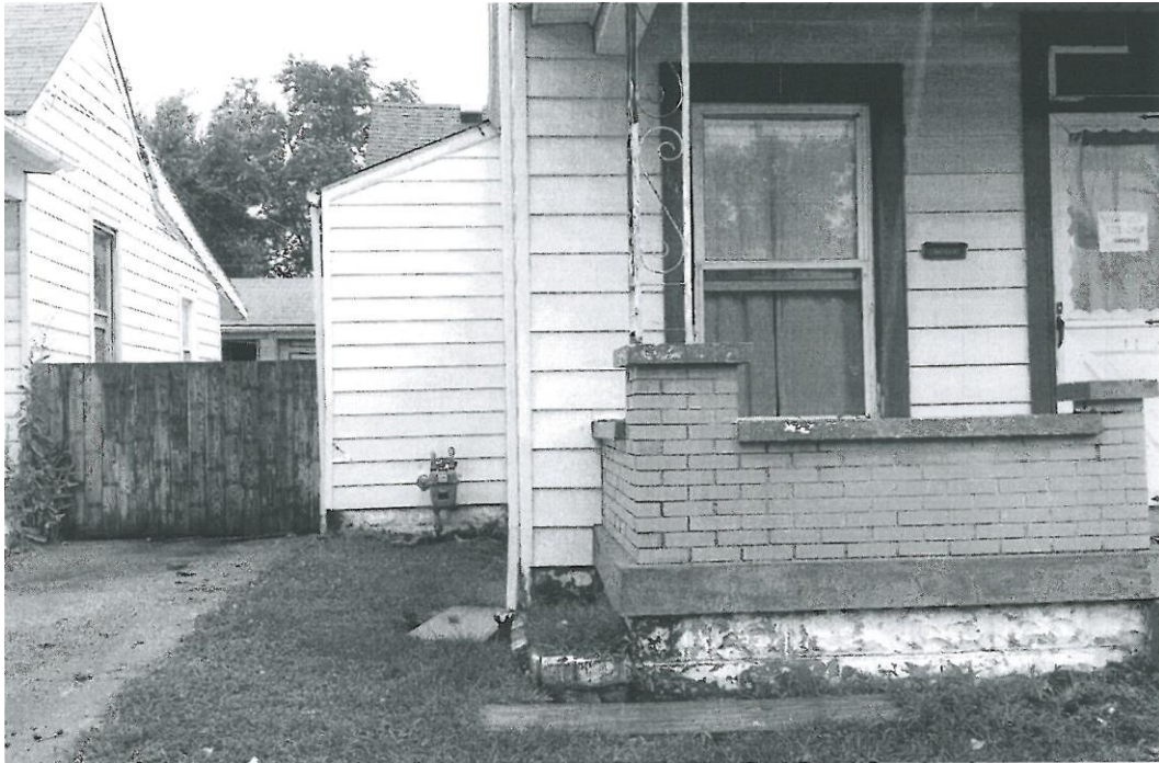
View of the existing SW side yard setback
