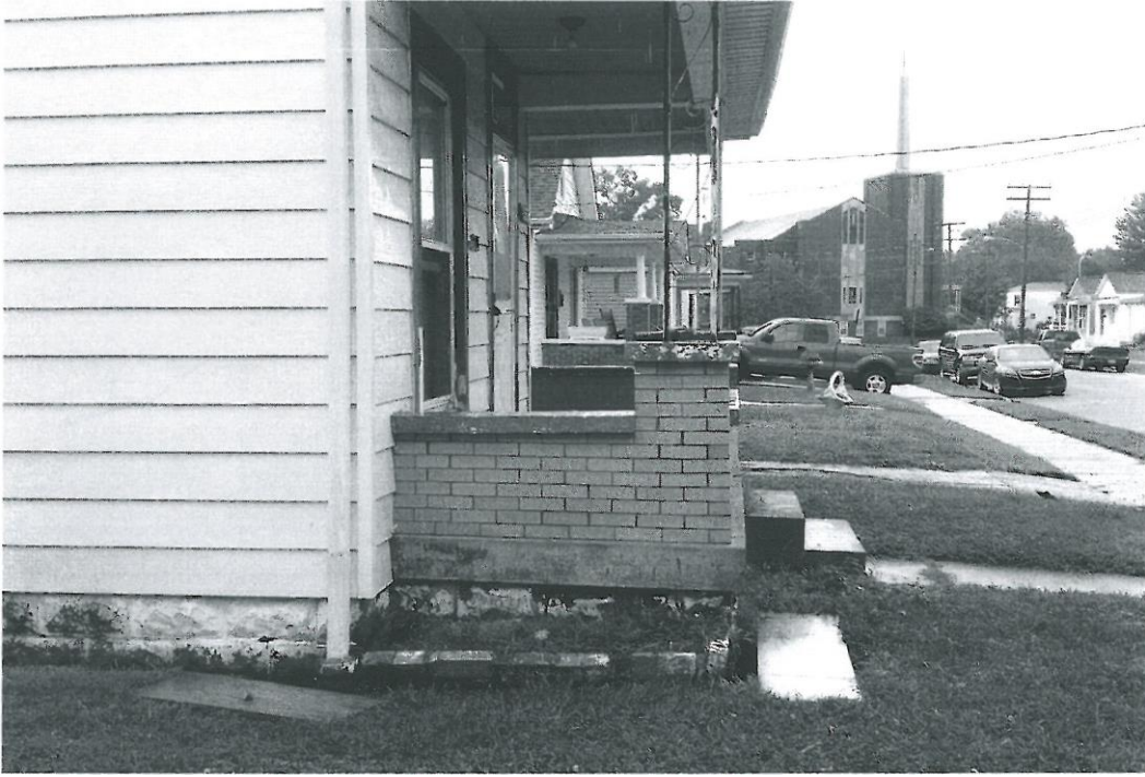
View of the front yard setbacks
