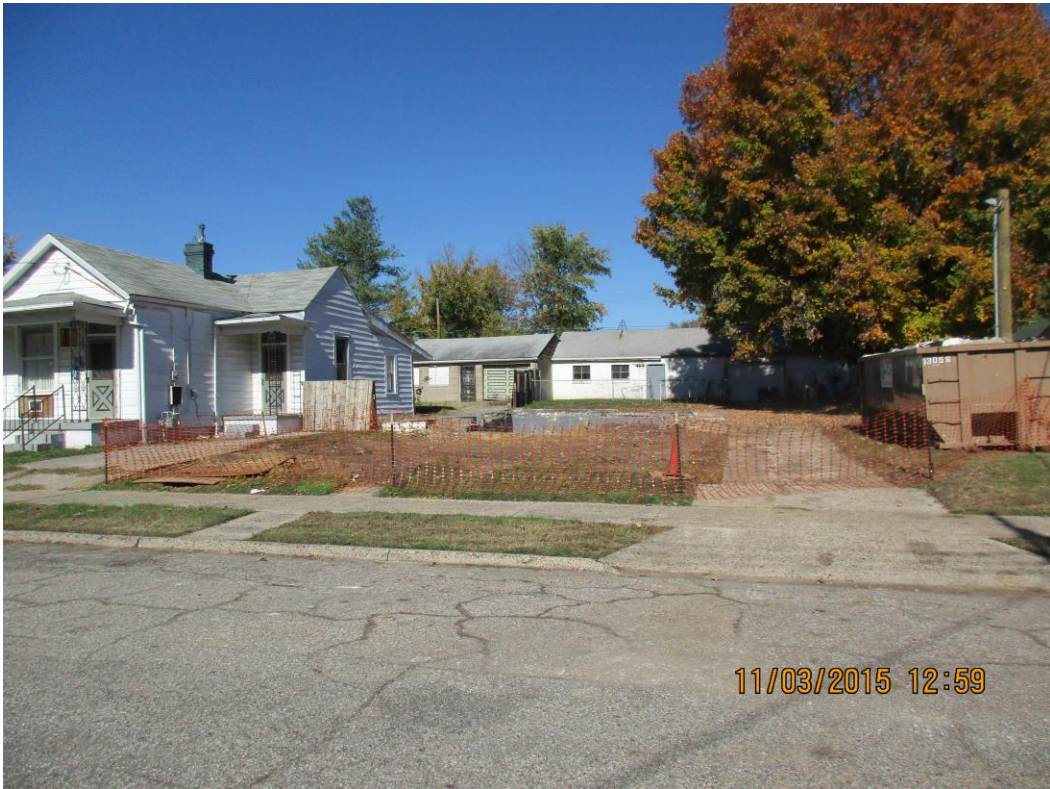
House has been removed
