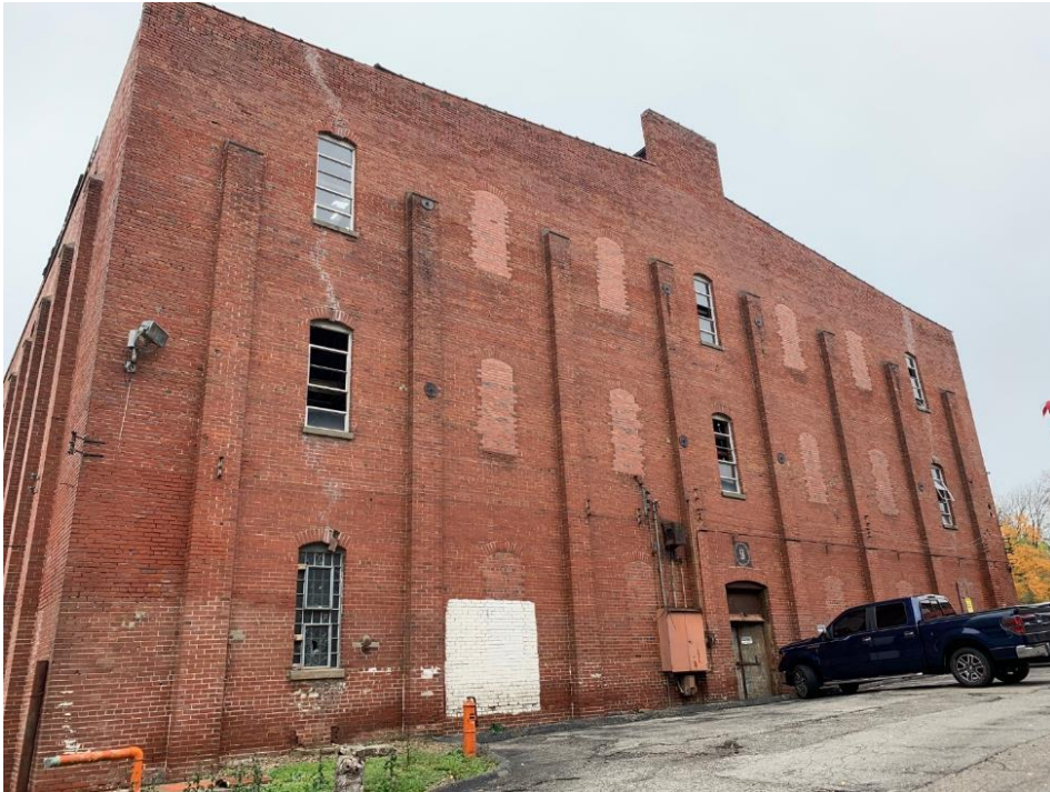
West Elevation (Staff Photo October 2020)
