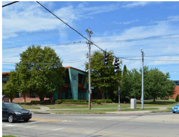
Mobility Recommendation 7: The intersection of Dutchmans Lane and Cannons Lane could be made more pedestrian-friendly with reduced corner radii, improved crosswalk markings, and a dedicated or early pedestrian signal phase.
