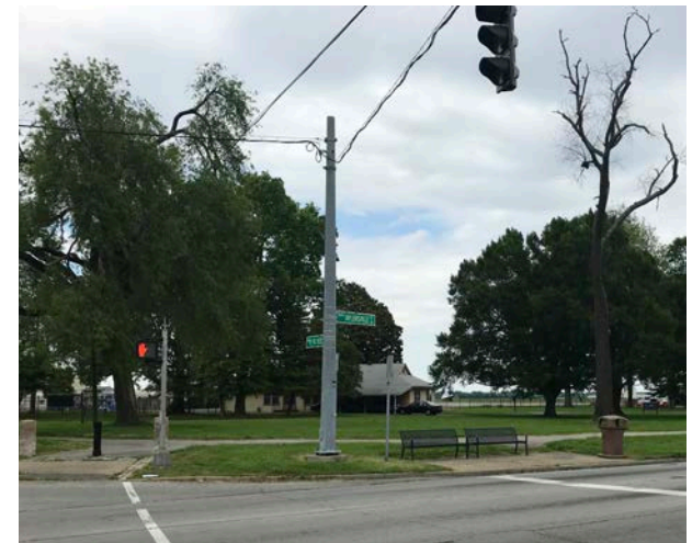
Mobility Recommendation 1: Another view of the same intersection. Additional pedestrian lighting and ADA accessible ramps would make the intersection safer and more inclusive.
