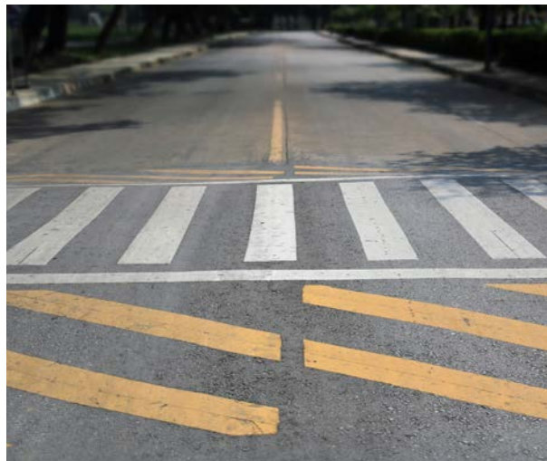
Mobility Recommendation 8: A speed table can be midblock or associated with a crosswalk, and is used to reduce traffic speeds.
