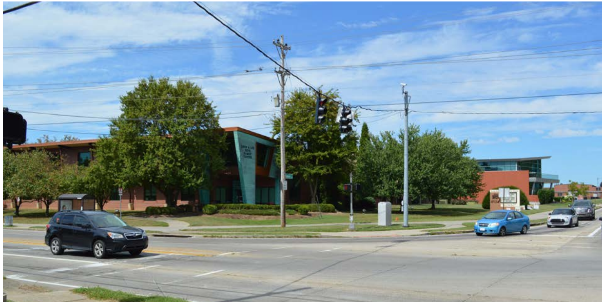
Mobility Recommendation 7: The intersection of Dutchmans Lane and Cannons Lane could be made more pedestrian-friendly with reduced corner radii, improved crosswalk markings, and a dedicated or early pedestrian signal phase.
