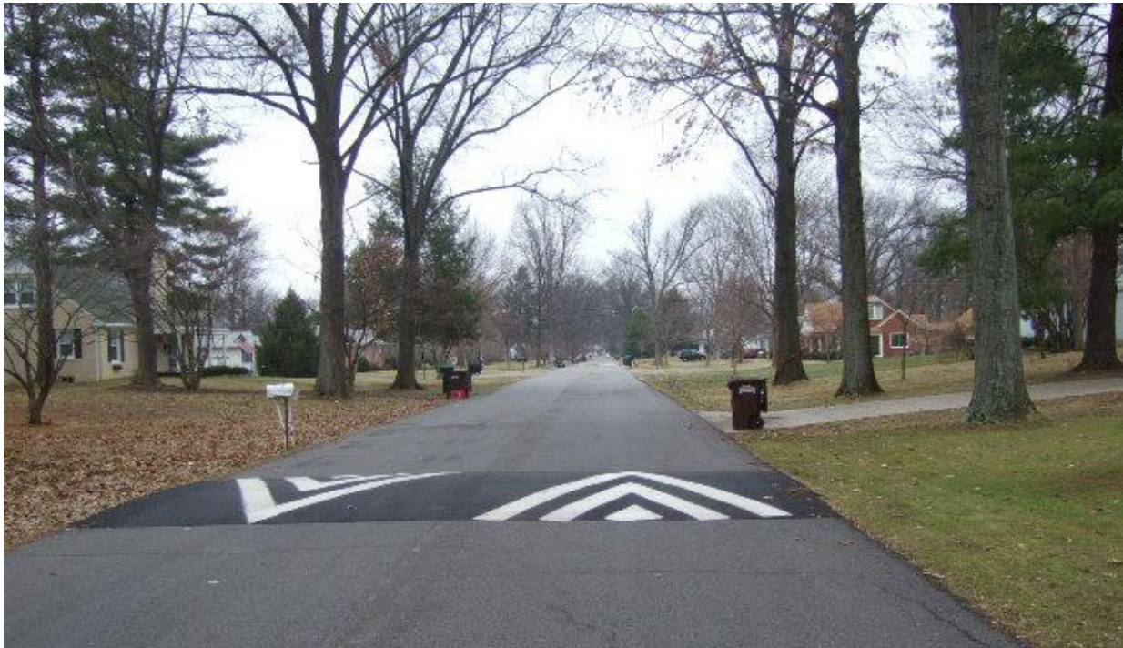
Mobility Recommendation 8: A speed hump is used to reduce traffic speeds.
