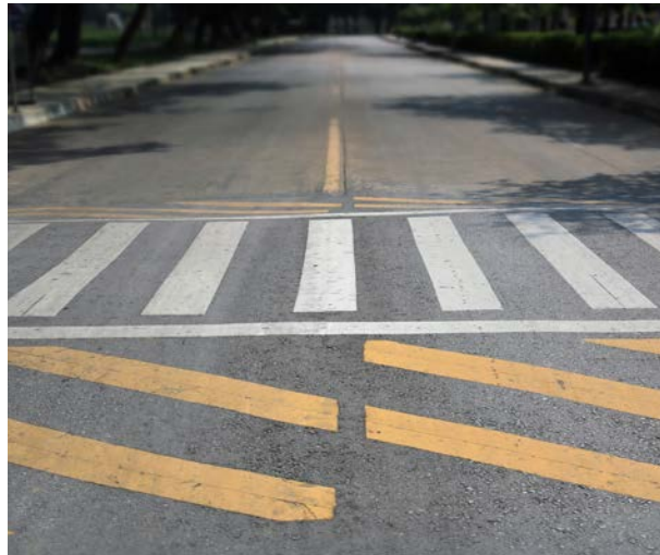
Mobility Recommendation 8: A speed table can be midblock or associated with a crosswalk, and is used to reduce traffic speeds.
