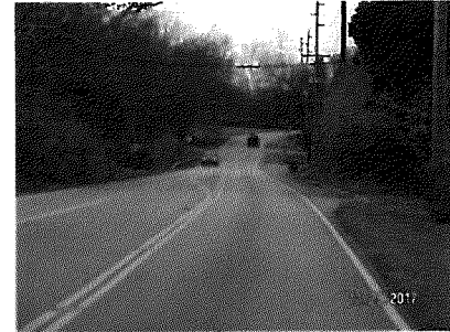
End Project – looking WB
