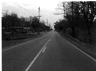
EB US 60 – location of cross drain (low point)
