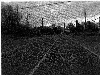
Begin Project – US 60 at Spring Drive
