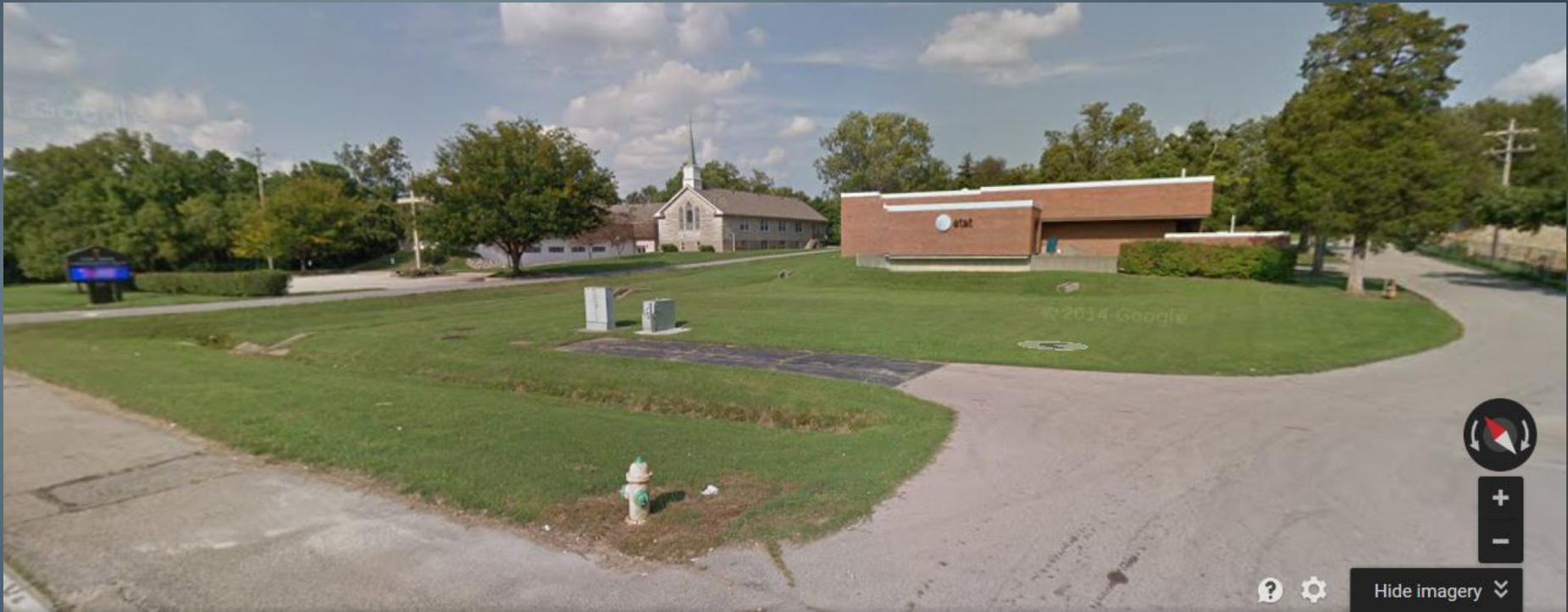
Looking north from AT&T facility (one building north of the new Raising Cane's restaurant) toward subject property.
