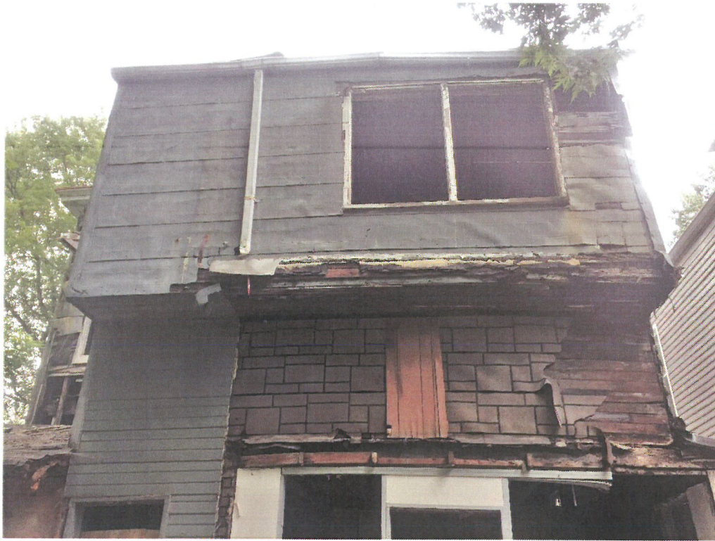
Photo 5 – View of the 2 nd Floor left side of the rear of the home. Note the deterioration of the 2 nd Floor framing on the overhang and lack of support structure on the 1 st Floor.
