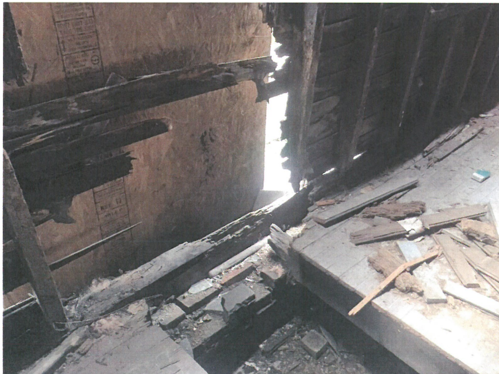
Photo 10 – Severe deterioration of the left side wall near the side door.
