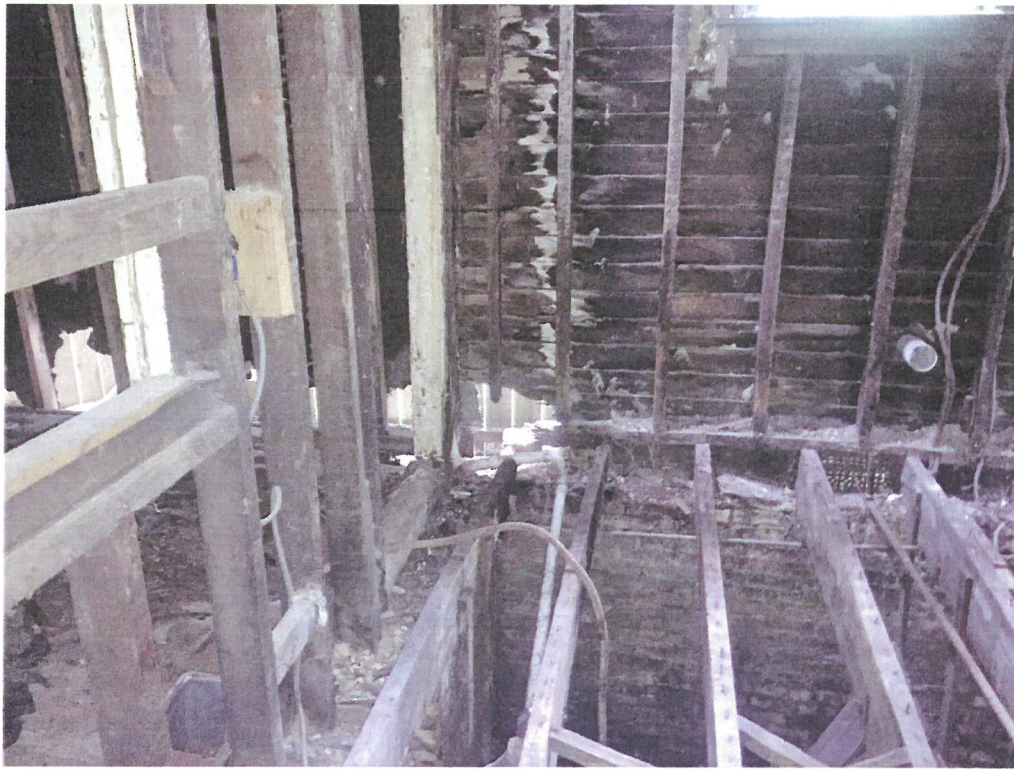
Photo 9 – Bottom of the right-side wall is rotted and missing. Ends of the joists are rotted as well.
