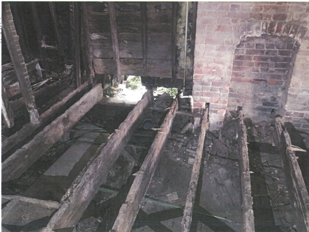
Photo 12 – More severe deterioration of the 1 st Floor joists and wall framing along the right wall in the front of the home
