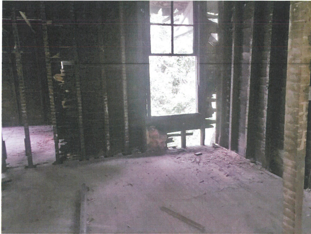
Photo 15 – View of the 2 nd Floor right rear corner deteriorated wall framing
