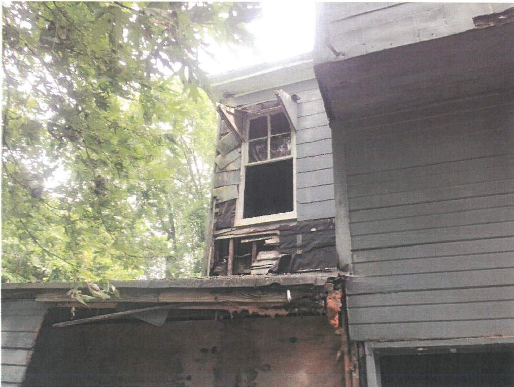
Photo 6 – View of the 2 nd Floor left side of the rear of the home. Note the severe deterioration of the wall framing and siding.
