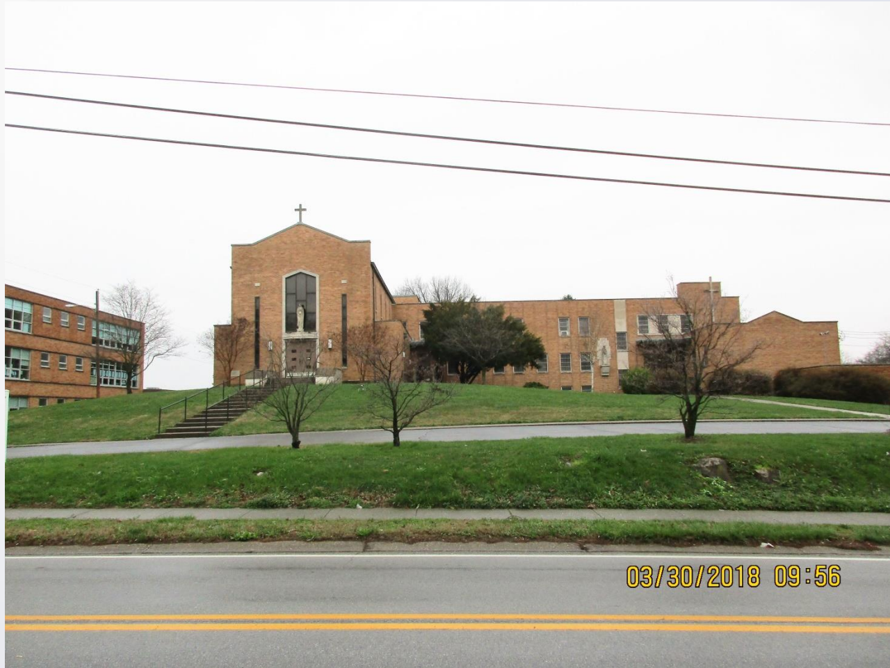
Street View of Convent Site
