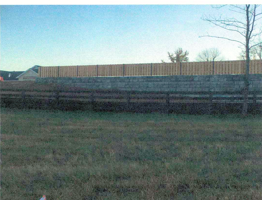
SITE PICTURE FROM I-265 RAMP
