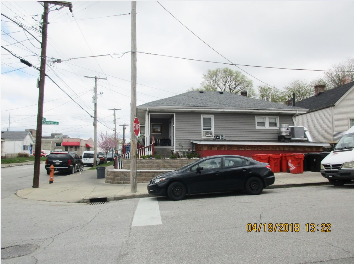
Adjacent to North (across Caldwell Street)
