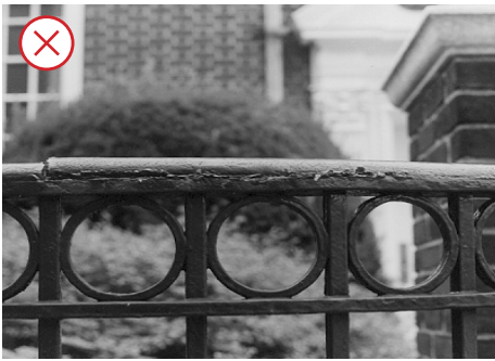
Clean a metal feature using appropriate techniques and materials so that the historic color, texture, or patina will not be damaged.
