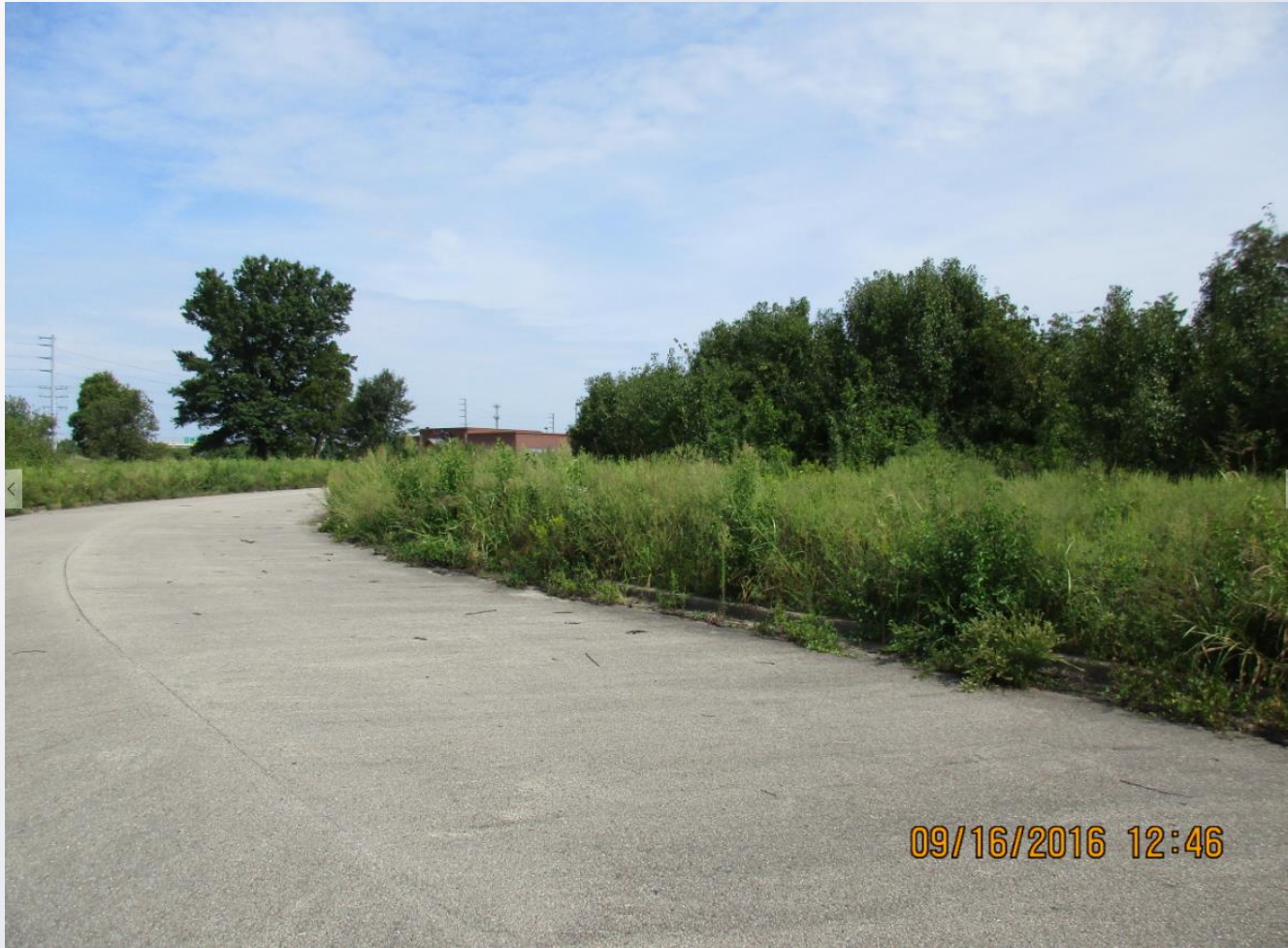
Site from Bullitt Lane looking northwest
