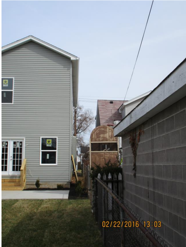
Looking Northeast at the rear of the property along the southern side of the property.
