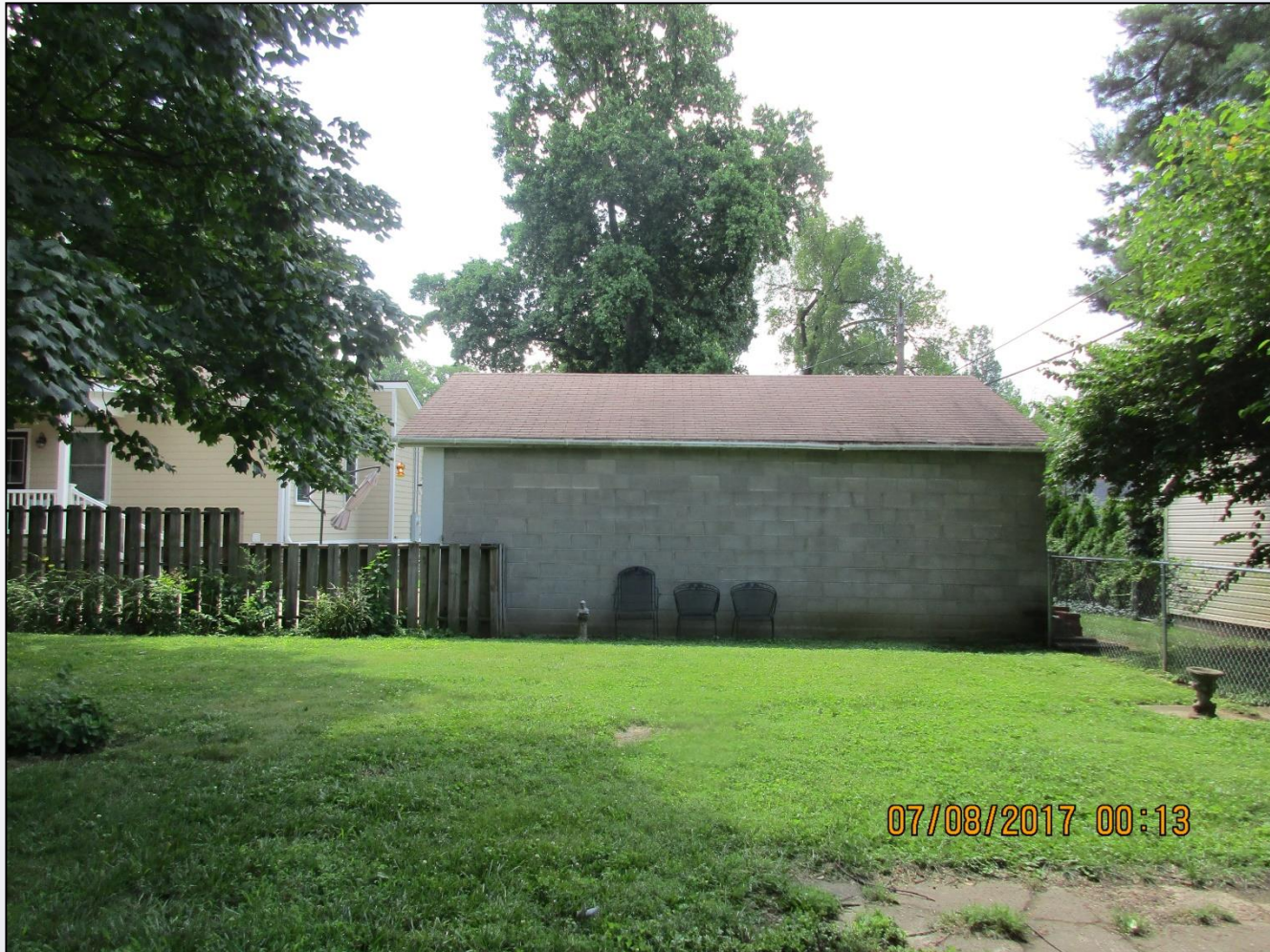
The existing garage on the property next door.
