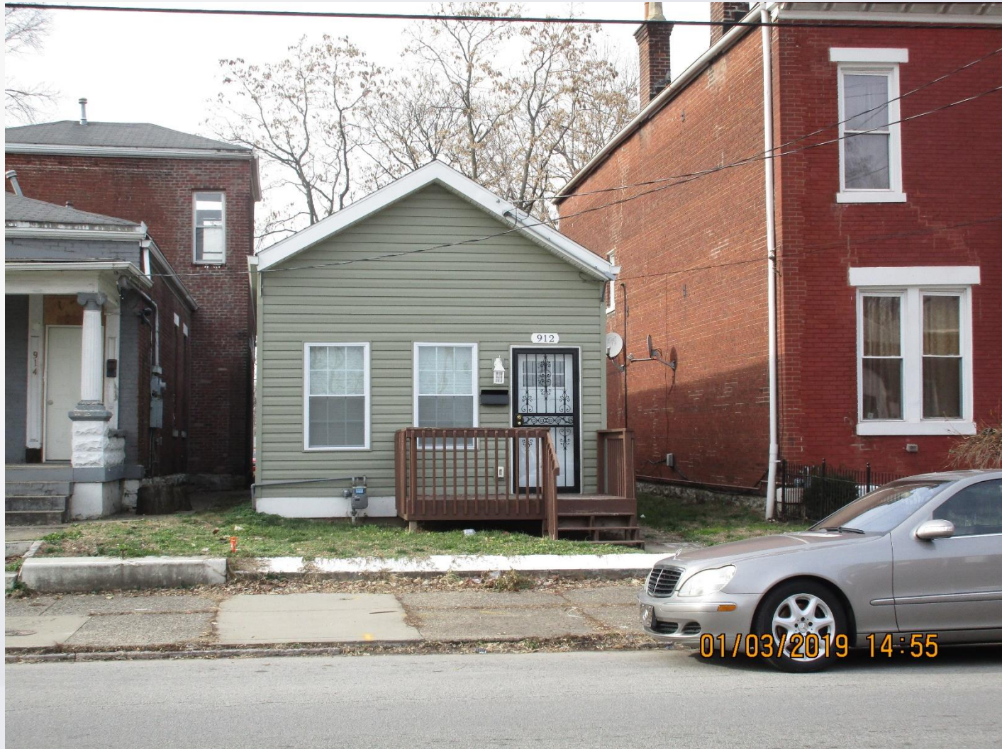
Adjoining Property to North
