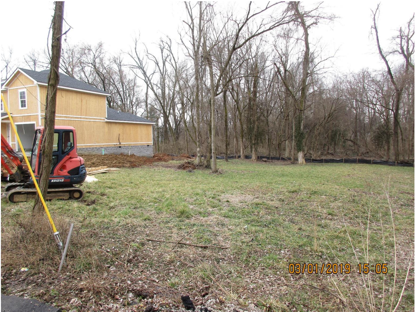
Property to the left of the subject property.
