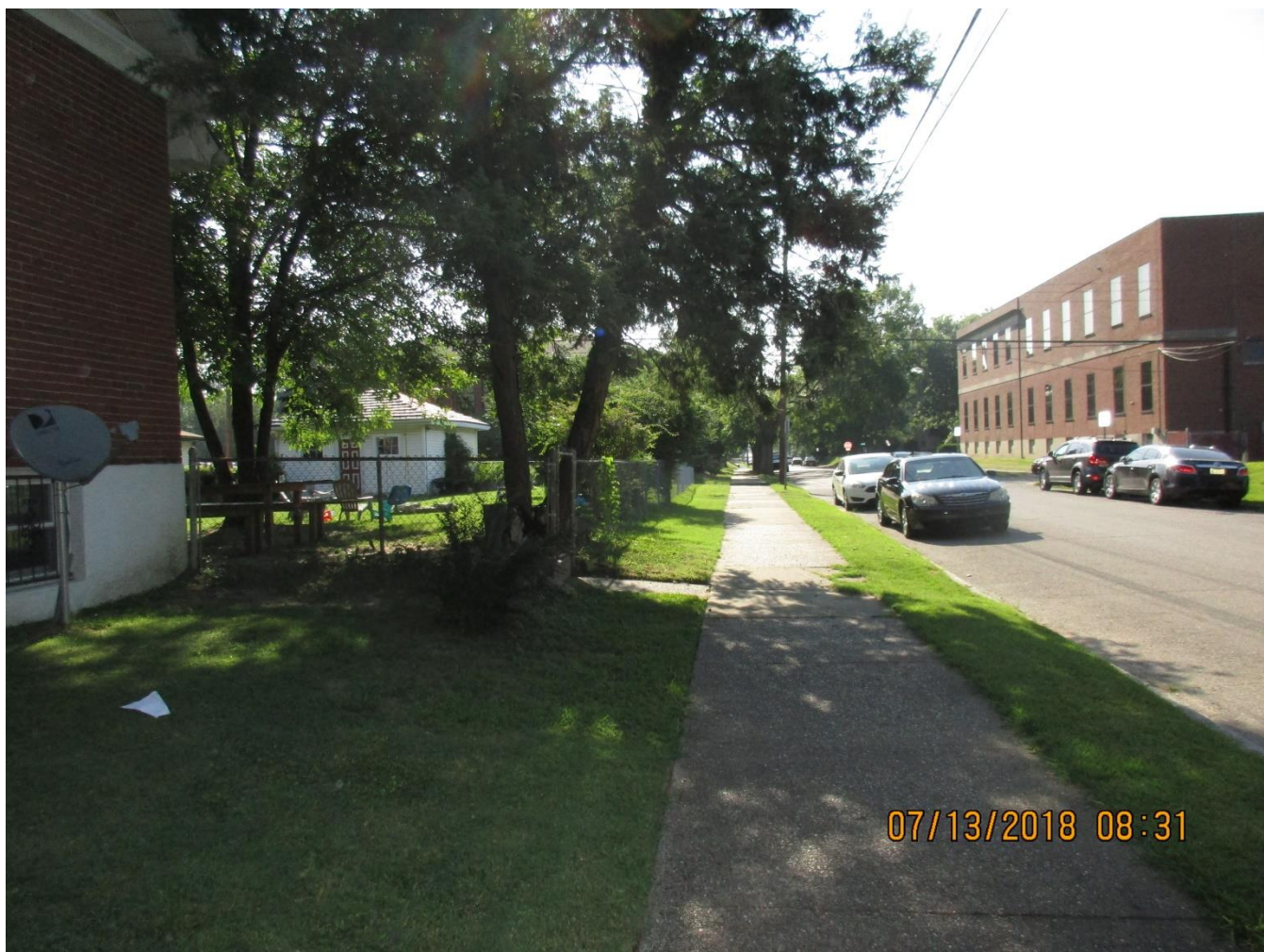
The existing fence to be replaced.
