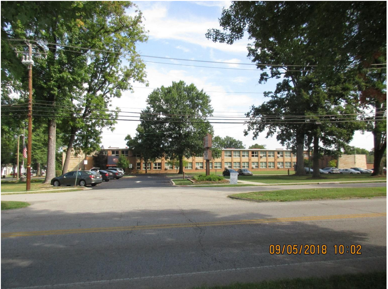
The front of the subject property with the sign to be replaced.
