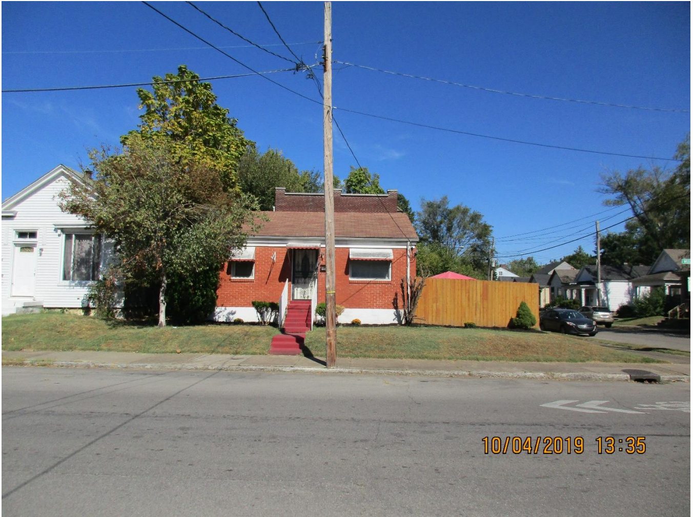
The property across Mulberry Street.
