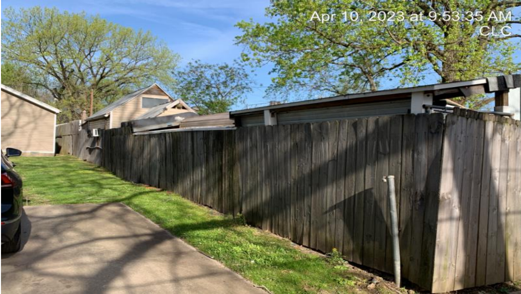
View of fence in the side yard setback.
