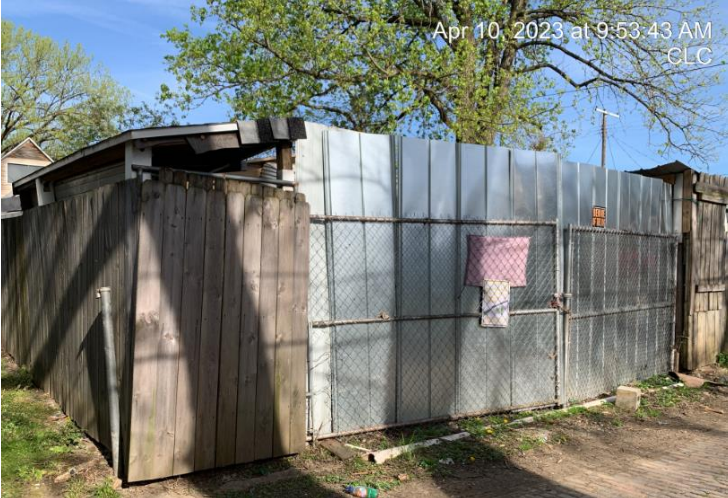
View of fence on rear property line.
