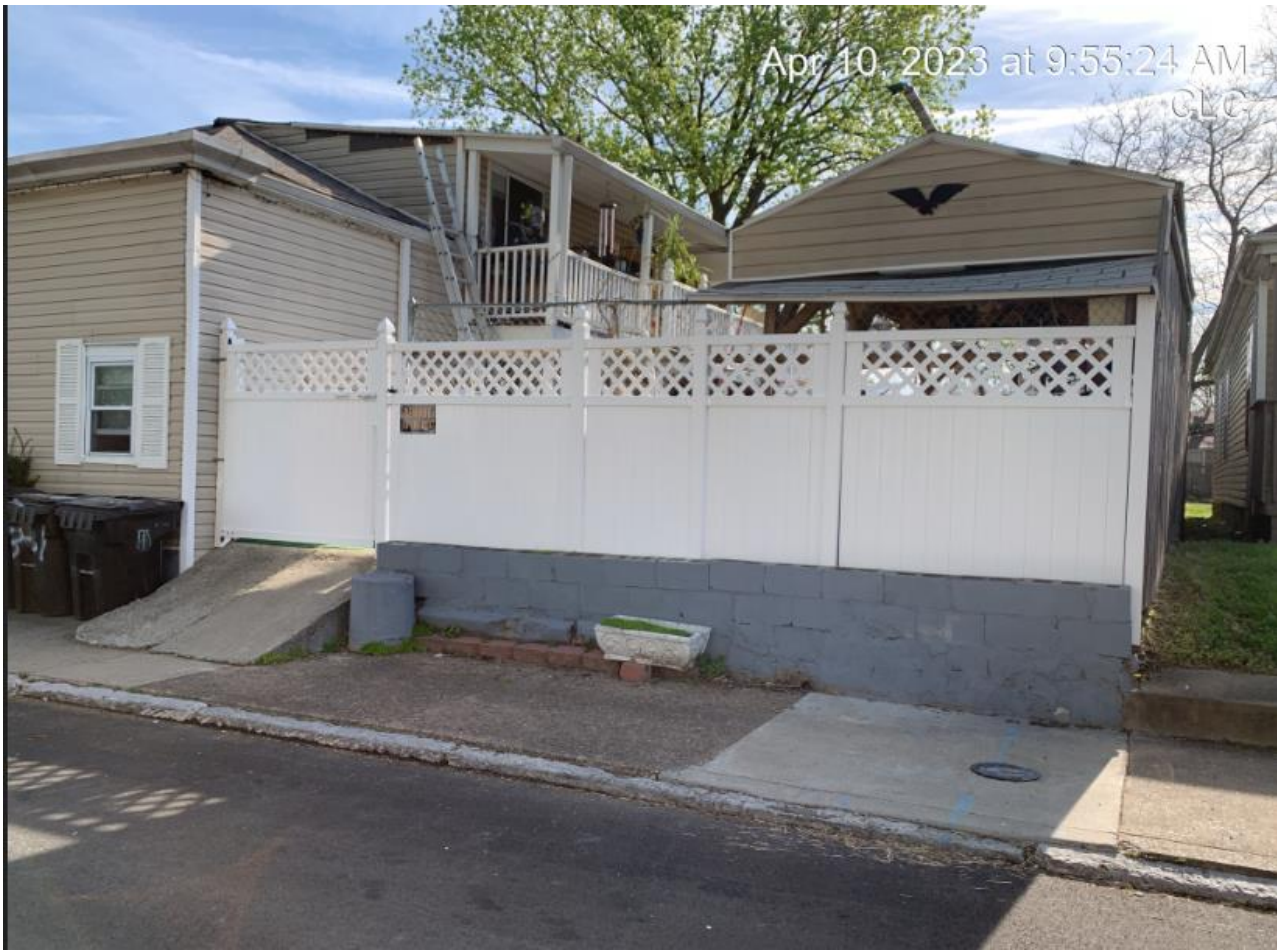
Front of subject property and fence in front yard setback
