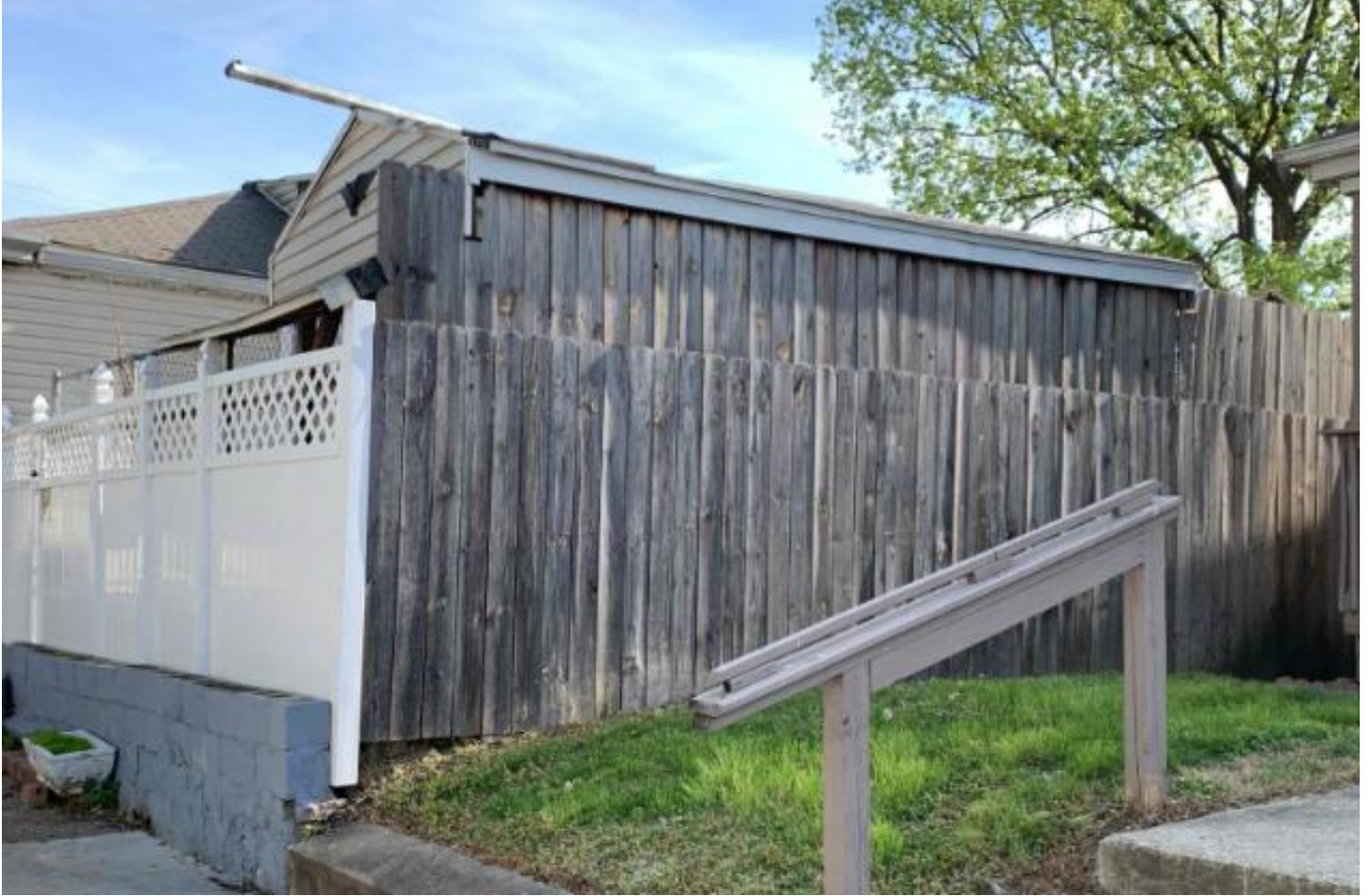
Fence in the side yard.
