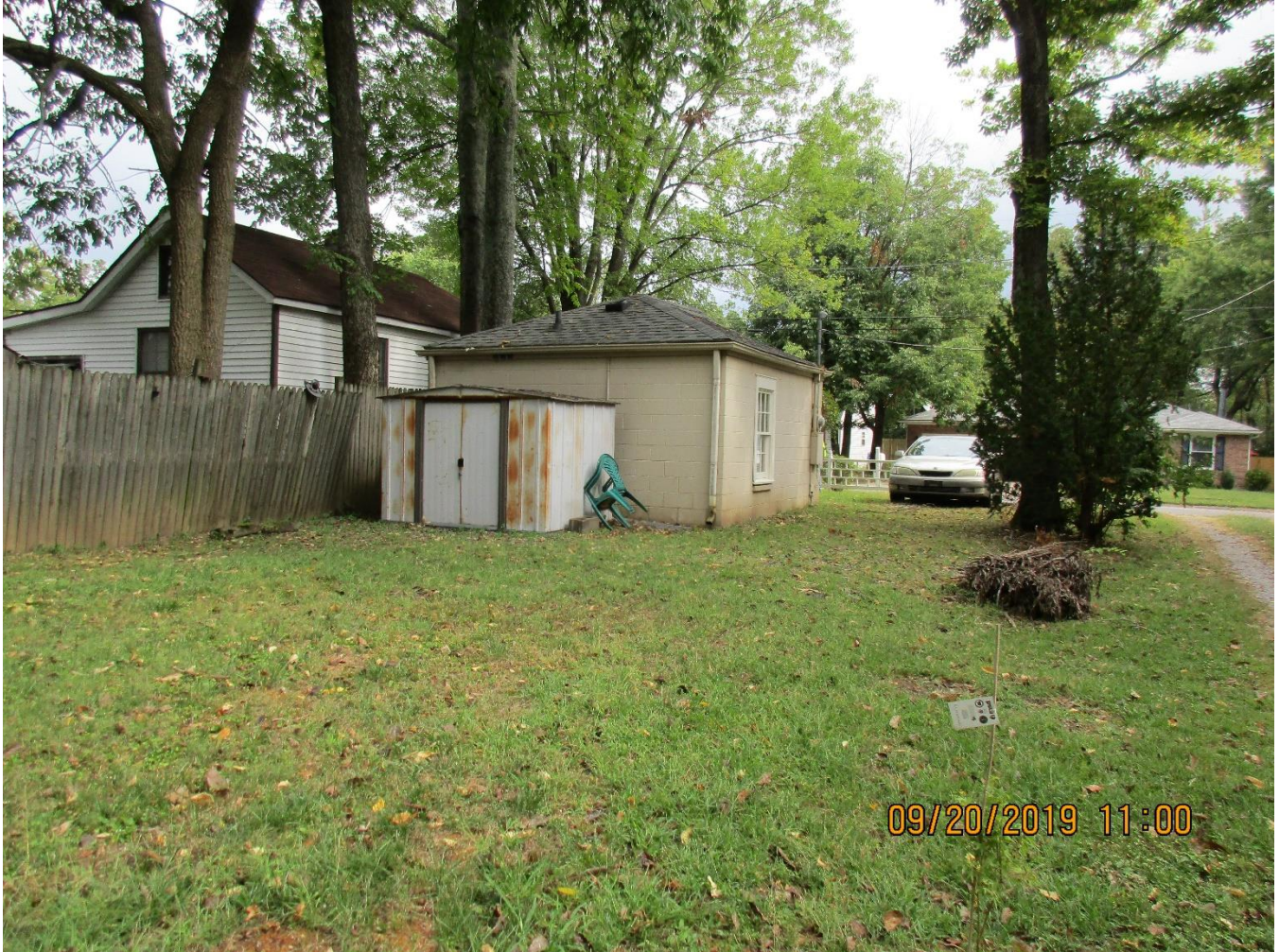
Existing structure from rear.
