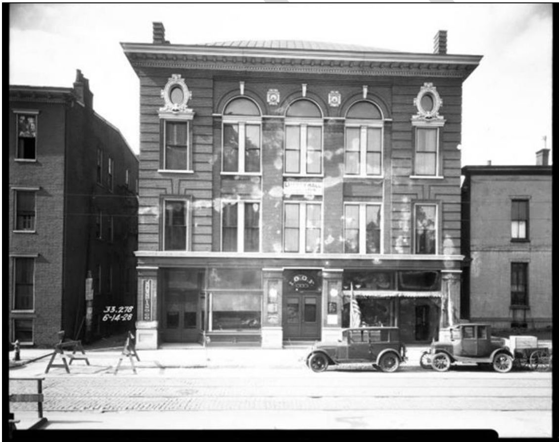
Figure 8. 1928 Metropolitan Sewer District Photograph of Liberty Hall.
