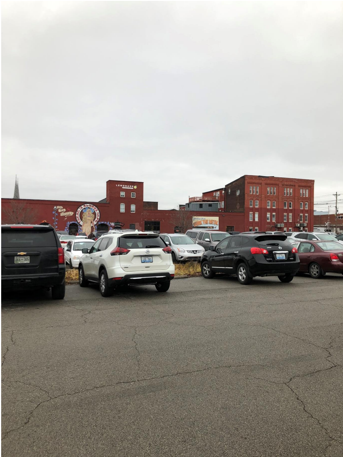
Western façade and location of existing signage.
