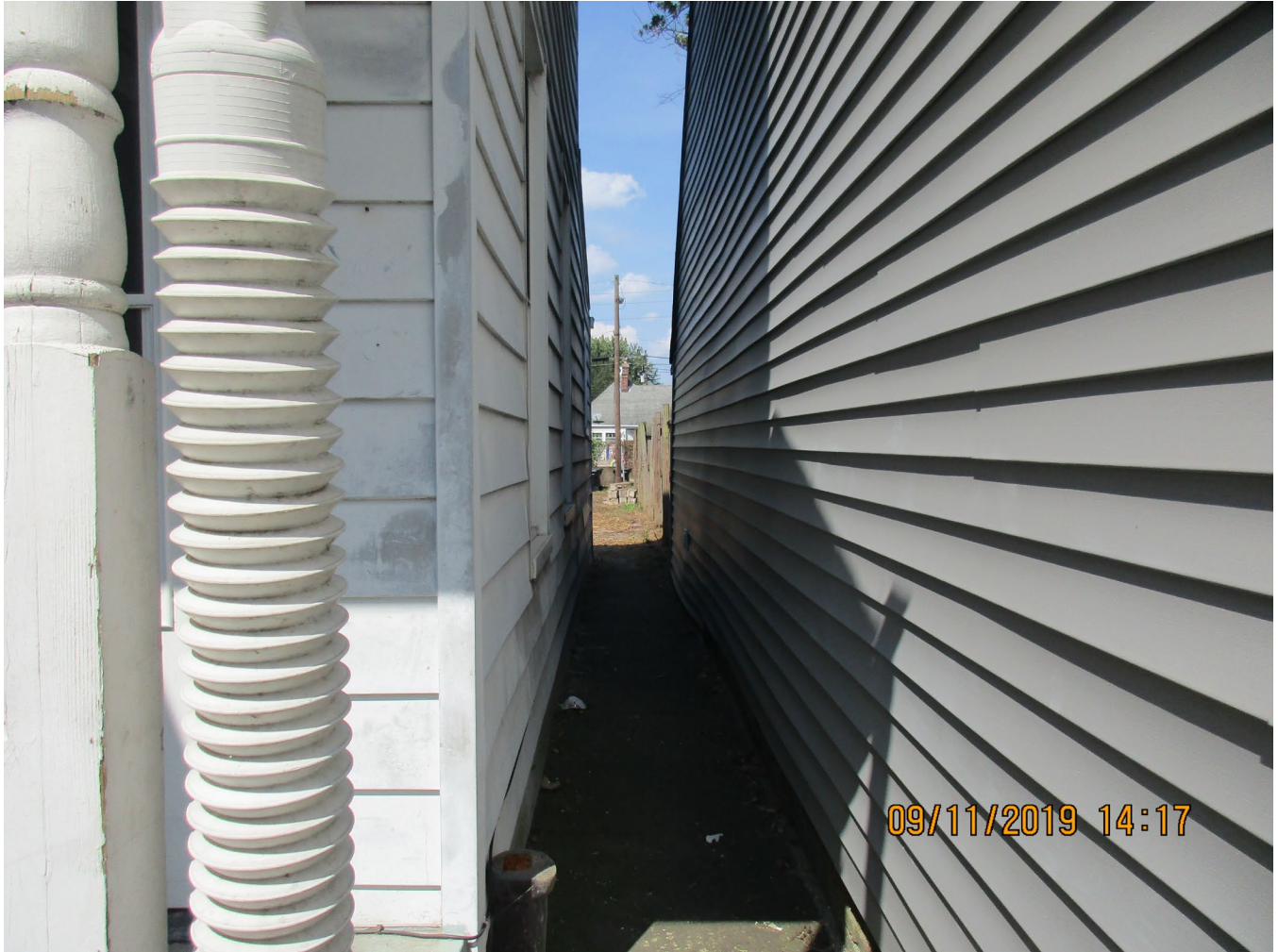
East side yard area.
