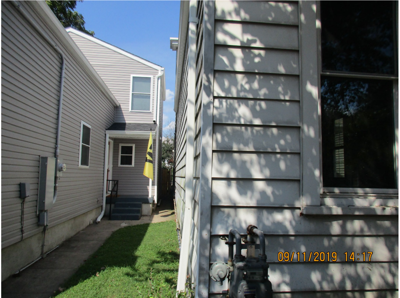
West side yard area.
