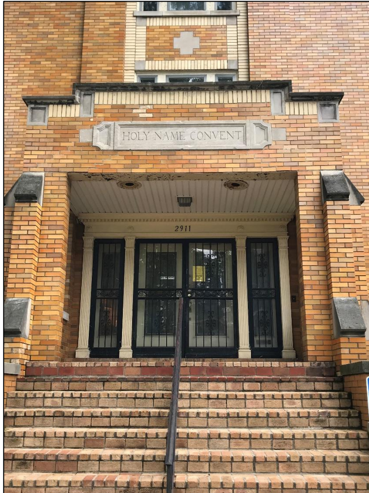
Figure 16. Front façade, or west elevation, detail of Building 4, looking east.
