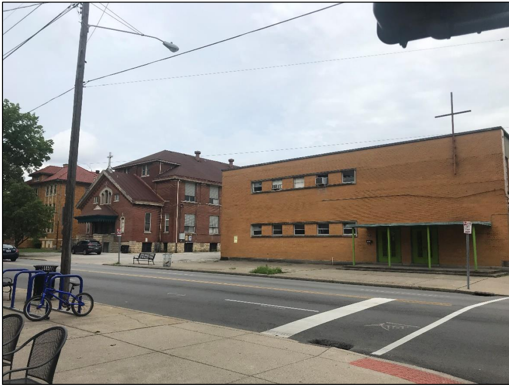
Figure 22. Photograph of S. Fourth Street showing Building 3, Building 4, and Building 5, looking northeast.
