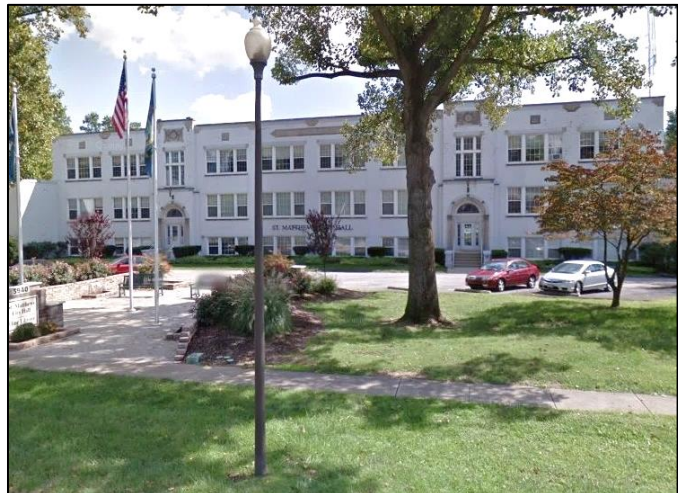
Figure 54. Greathouse School, 3940 Grandview Avenue (Google)
