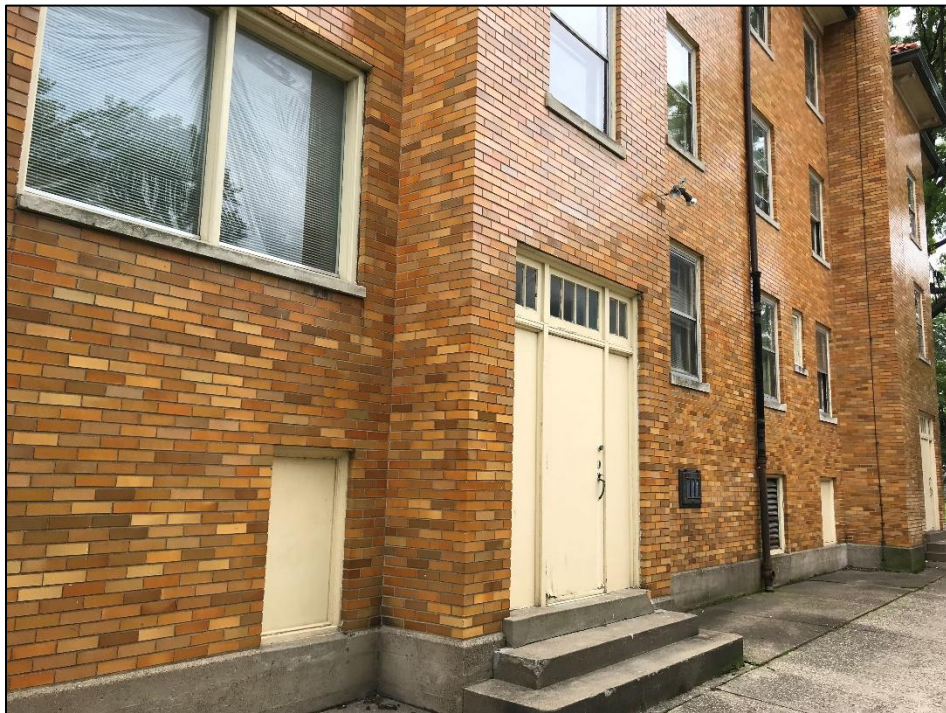
Figure 21. North elevation of Building 4, looking southwest.
