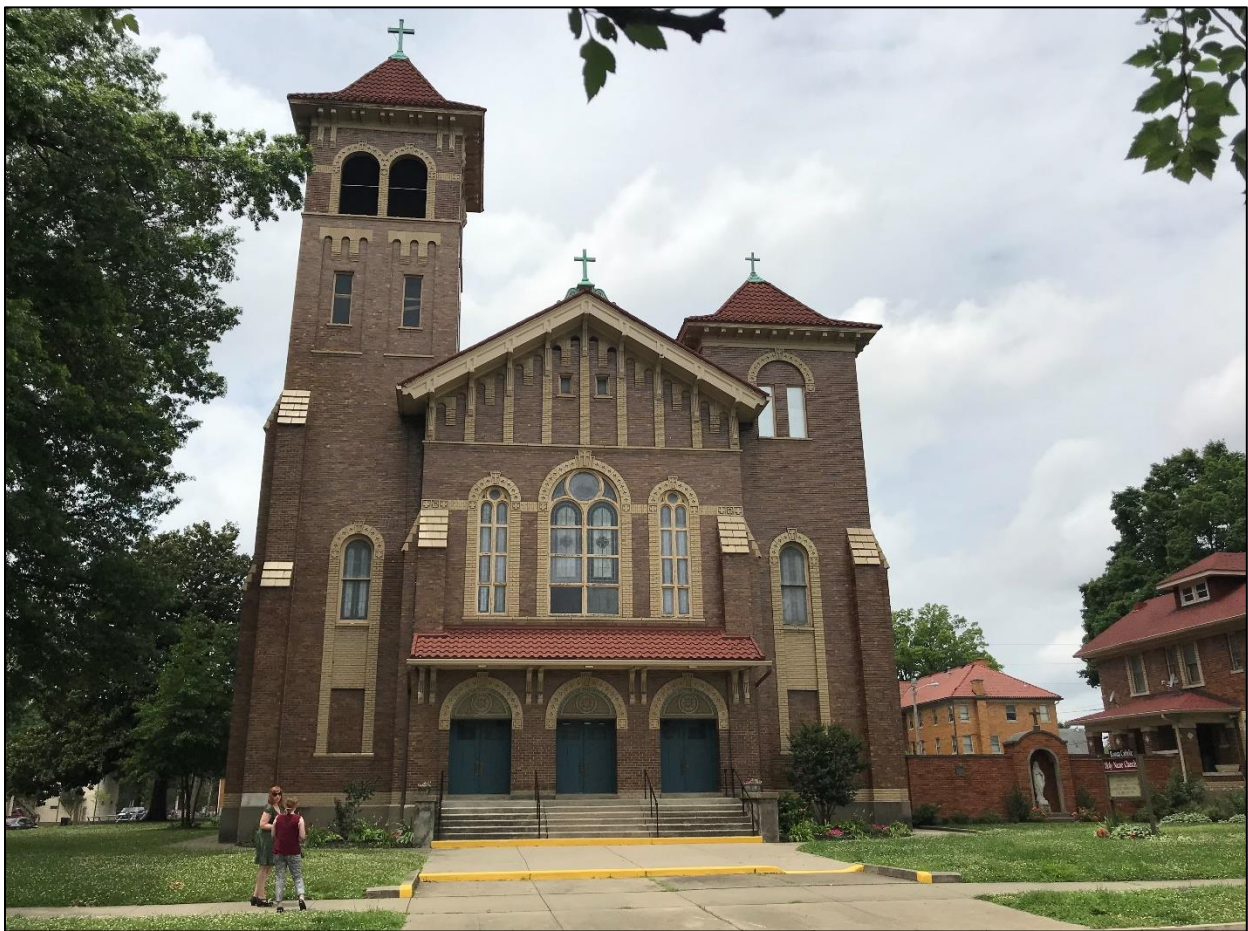
Figure 2. Front façade, or east elevation, of Building 1, the Holy Name Church, looking west.
