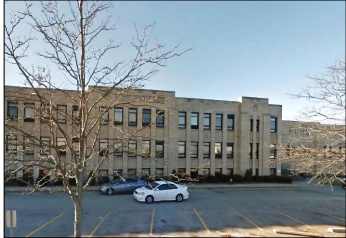
Figure 55. Fern Creek High School, 9115 Fern Creek Road (Google)
