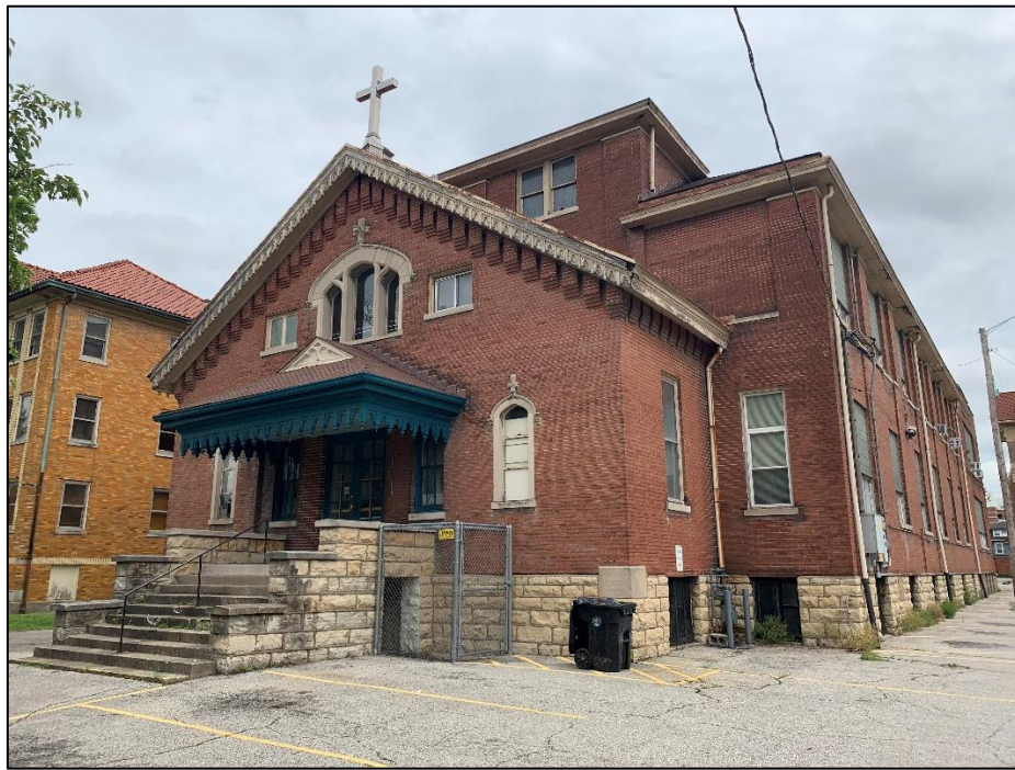
Figure 11. Front façade, or west elevation, of Building 3, the School, looking northeast.
