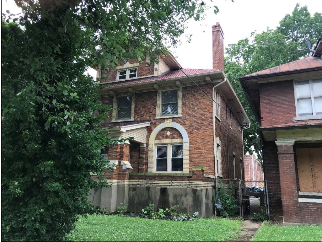
Figure 9. East and north elevations of Building 2, looking west.
