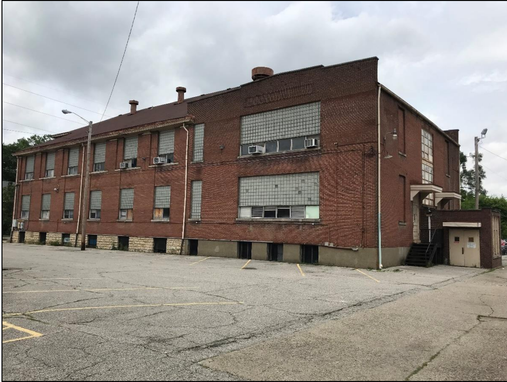
Figure 13. South elevation of Building 3, looking northwest.
