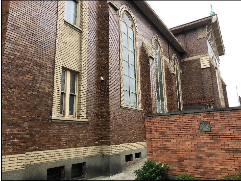
Figure 4. North elevation of Building 1, looking southwest.
