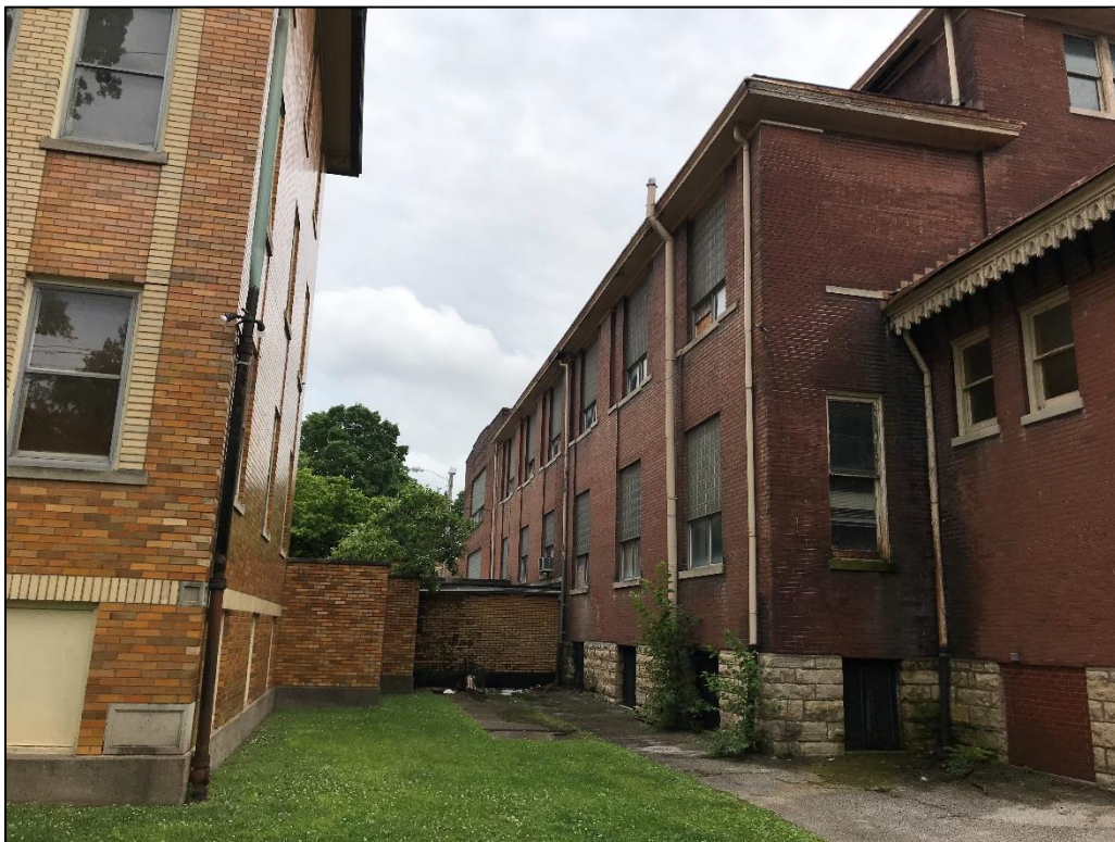
Figure 14. West and north elevations of Building 3, looking east.
