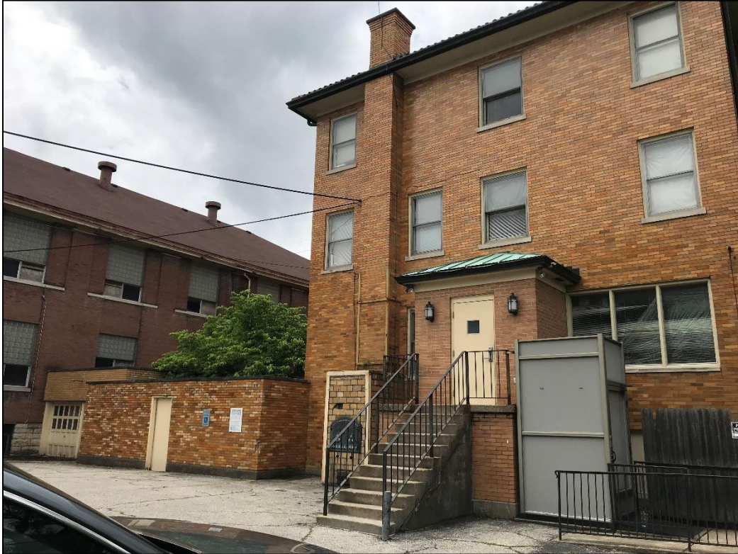
Figure 18. East, or rear, elevation of Building 4, looking southwest.
