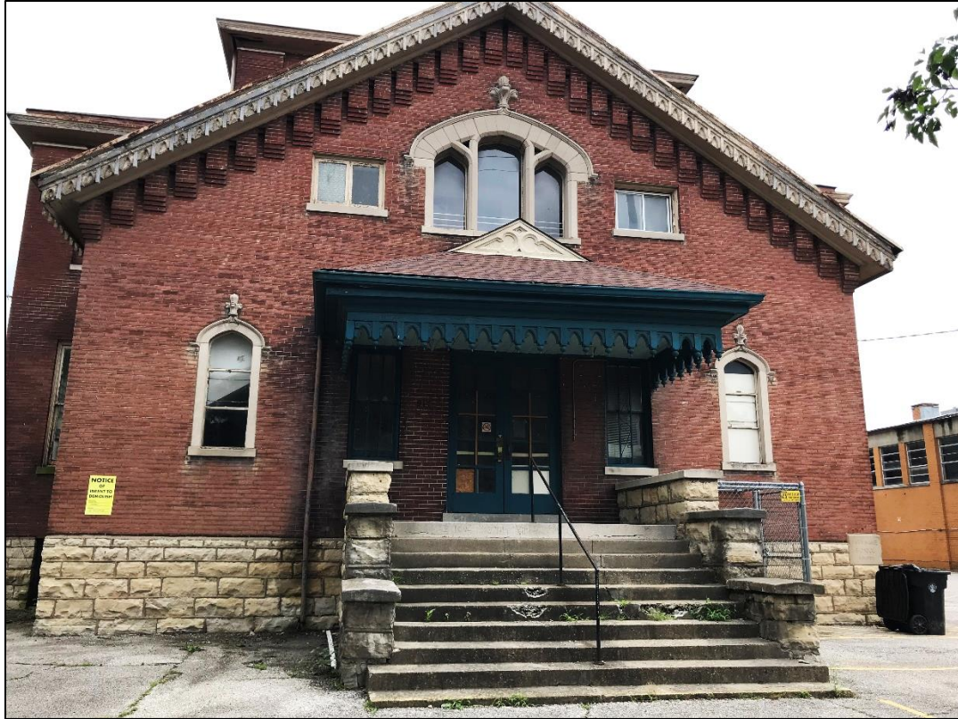
Figure 12. Front façade, or west elevation, of Building 3, the School, looking east.
