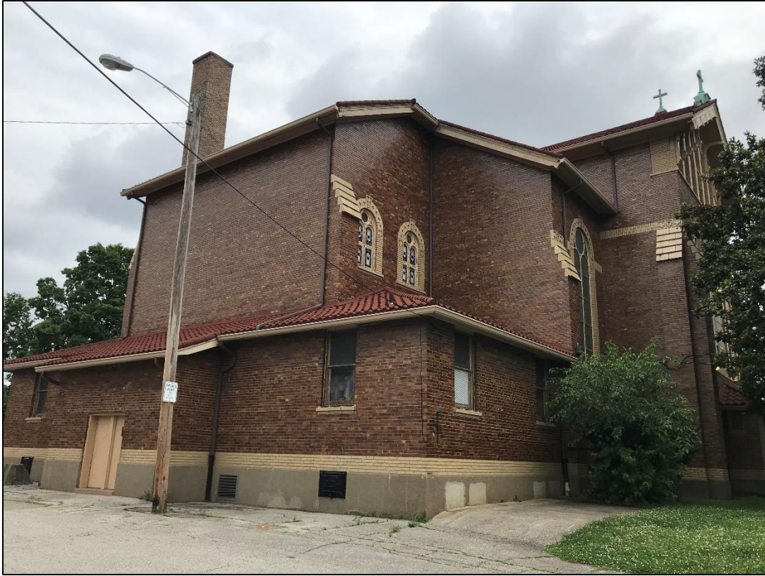
Figure 7. West, or rear, elevation of Building 1, looking northeast.
