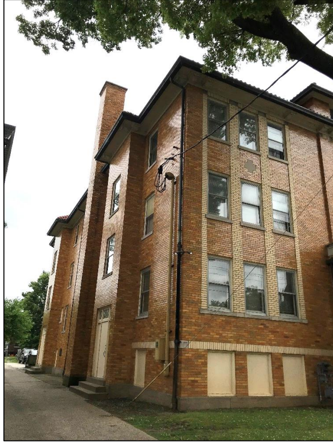
Figure 20. North and west elevations of Building 4, looking southeast.
