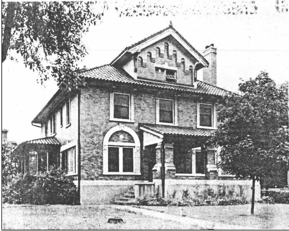
Figure 32. 1941 photograph of the Rectory Building designed by James J. Gaffney, known as Building 2 (Holy Name Parish 1941).
