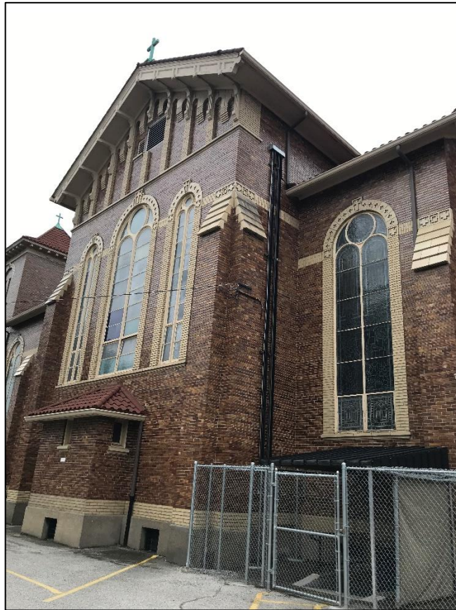
Figure 5. North elevation of Building 1, looking southeast.
