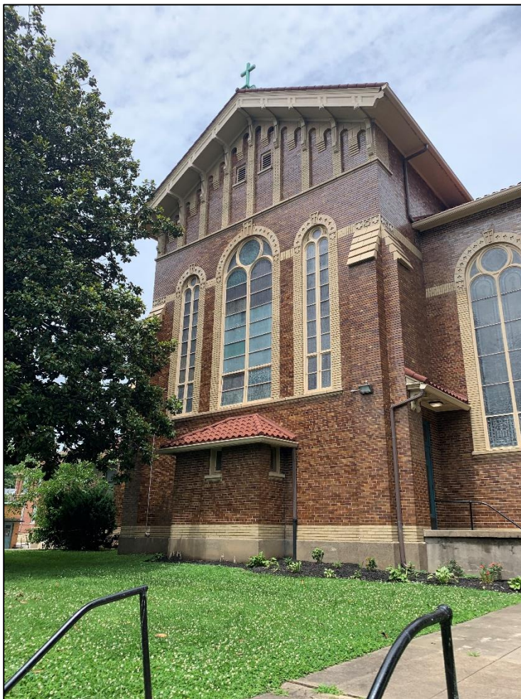
Figure 6. South elevation of Building 1, looking northwest.
