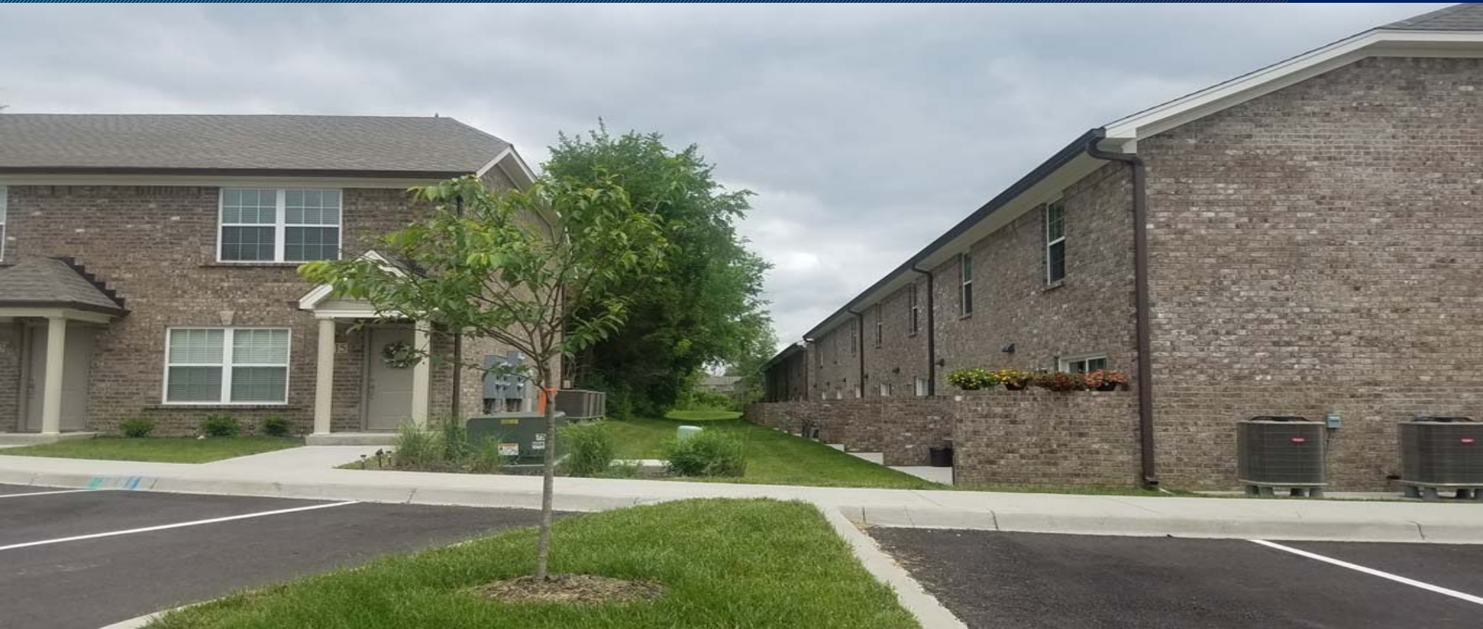
Similar style and design of townhomes built at Avalon Springs, on Beulah Church Road.
