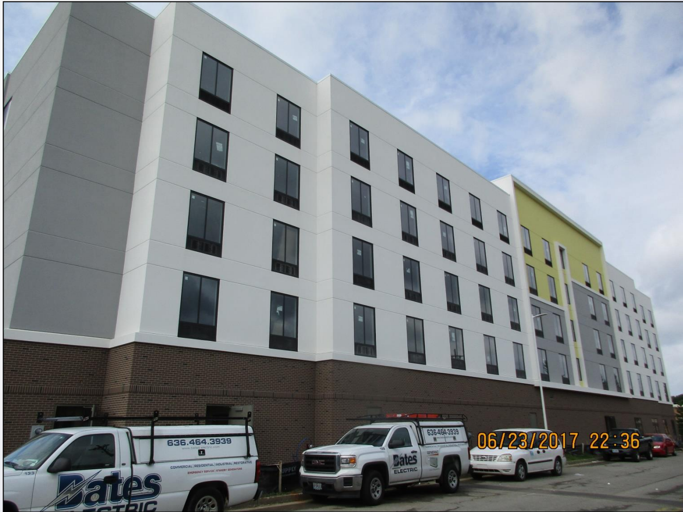
The north façade of the hotel.
