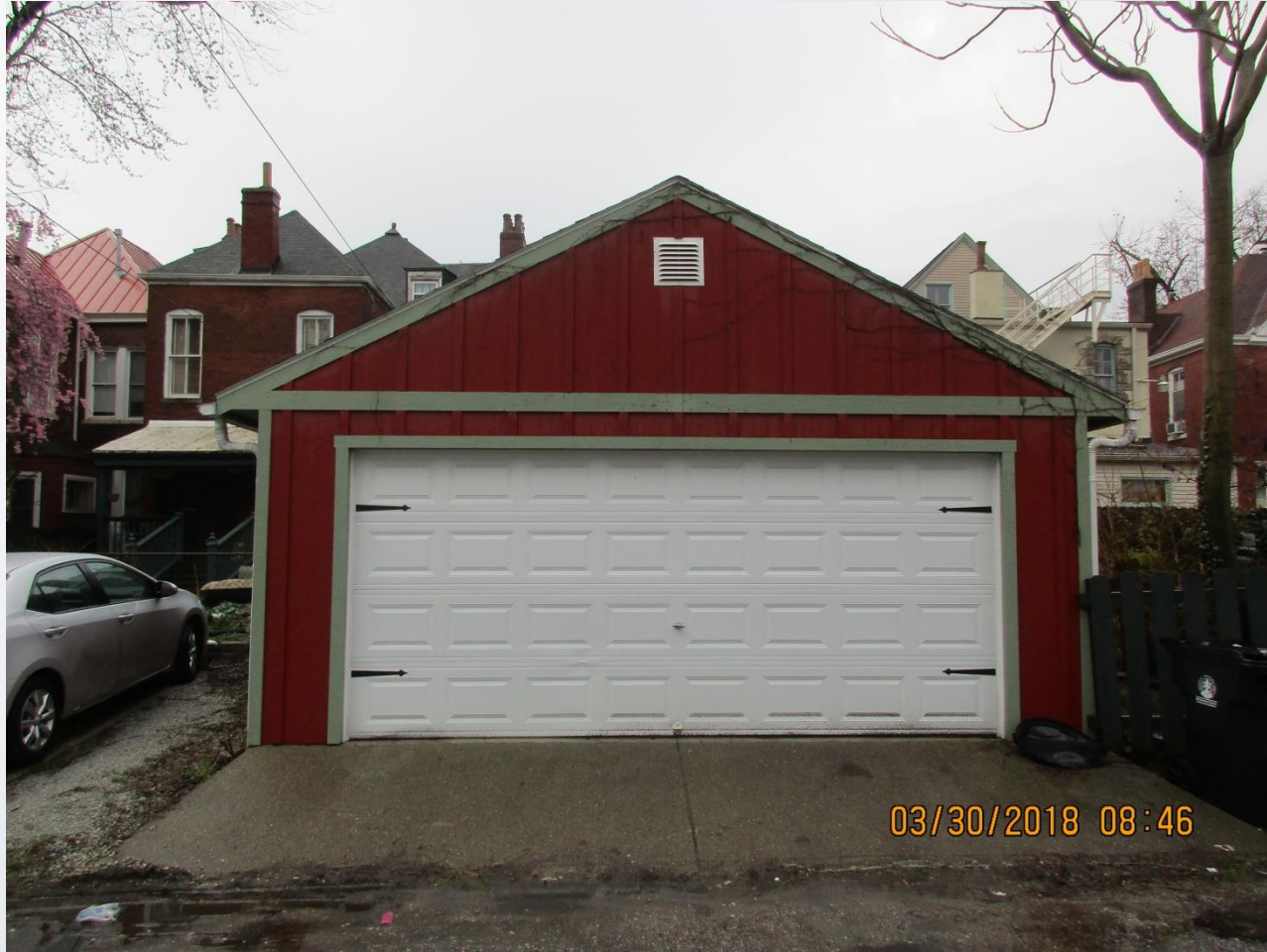
Garage at Rear Alley
