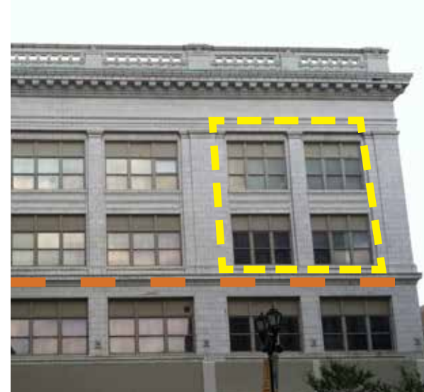
Brick or stone masonry & distinct base condition
