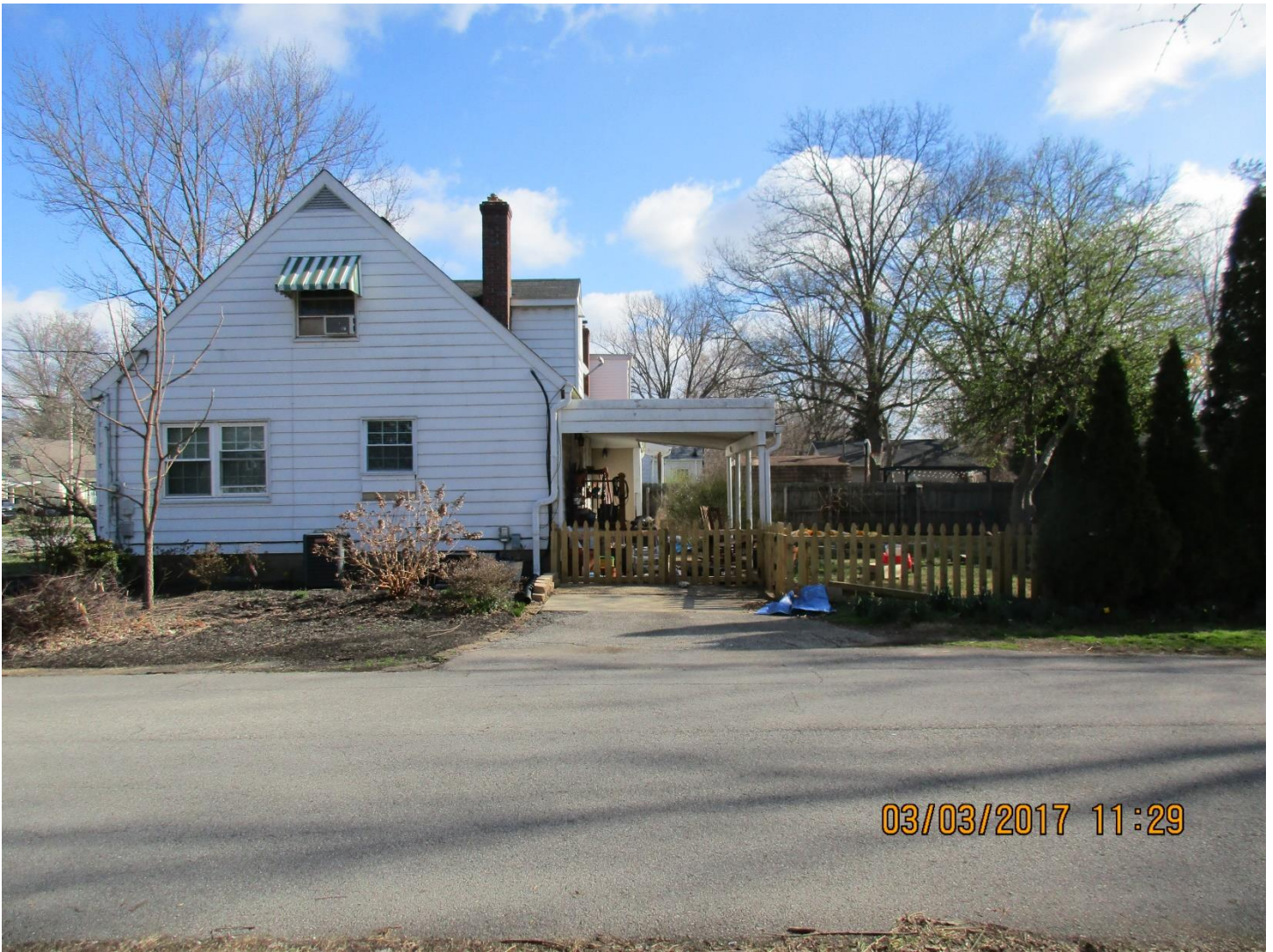
The side of the house where the addition is proposed.
