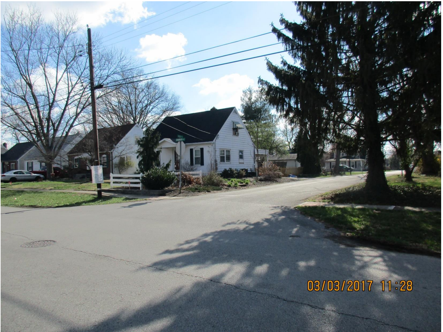
Looking at the side of the house where the addition is proposed.
