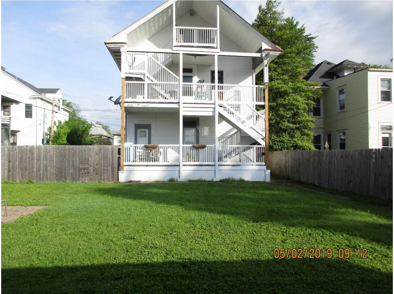
Private yard area looking toward the principal structure.
