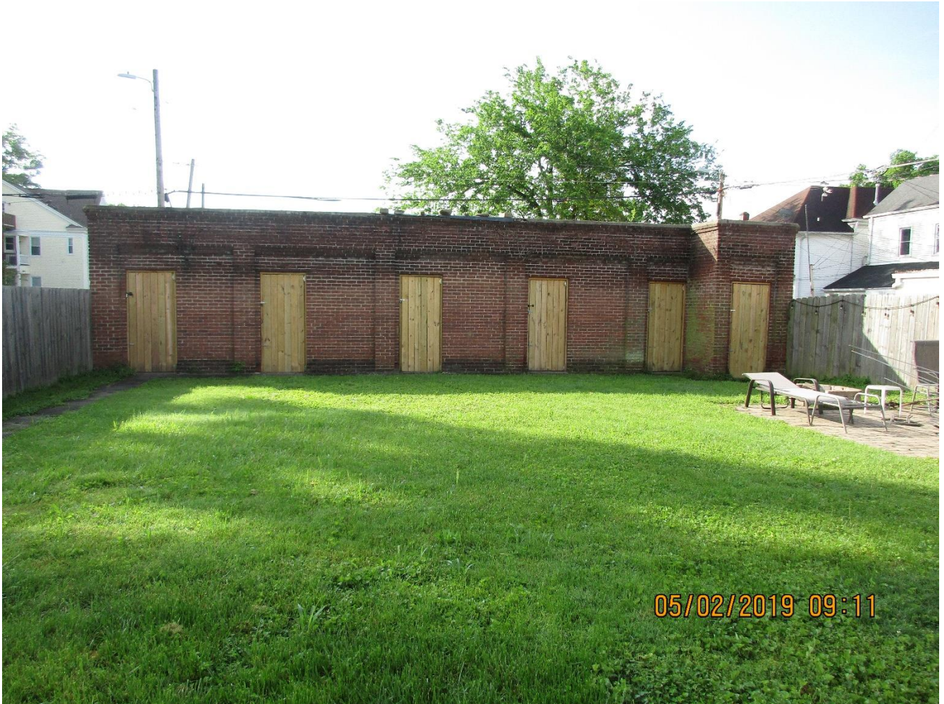
Existing private yard area.
