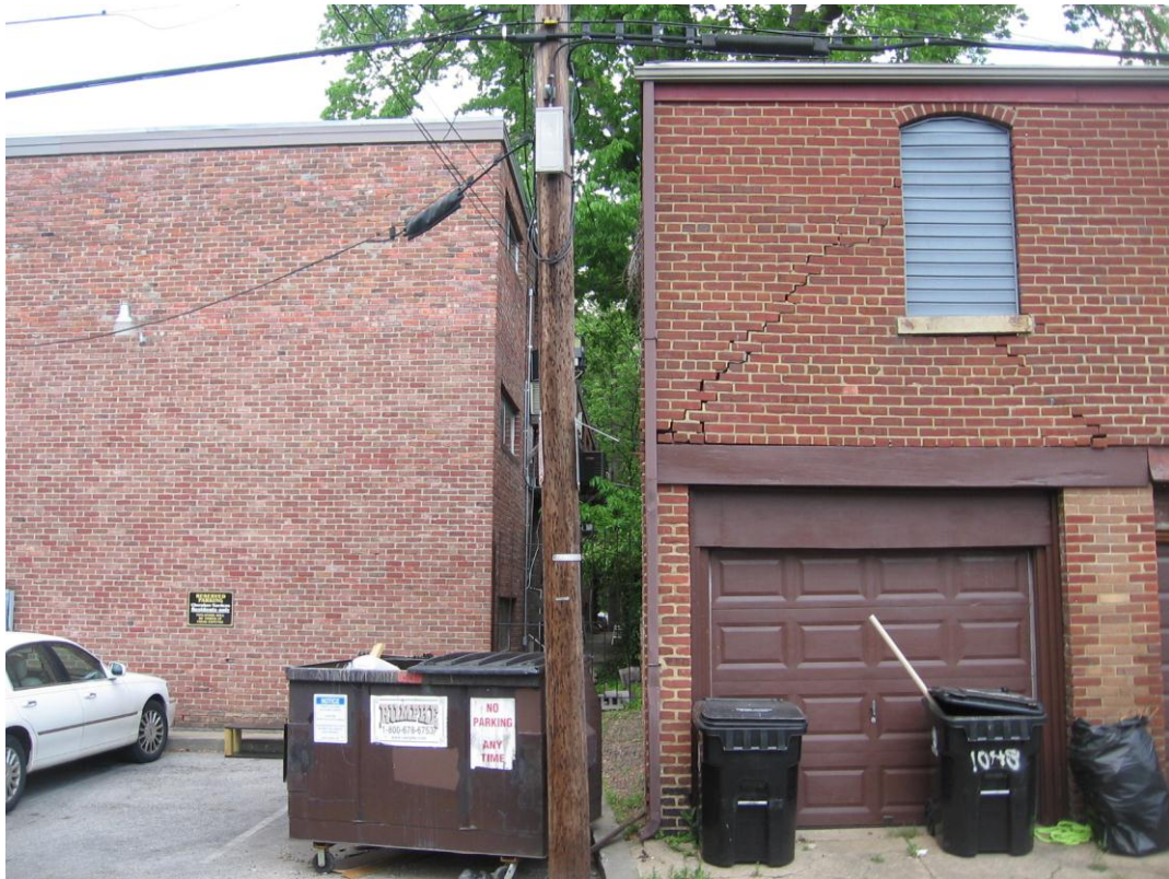
Rear of carriage house /northwestern perimeter of property
