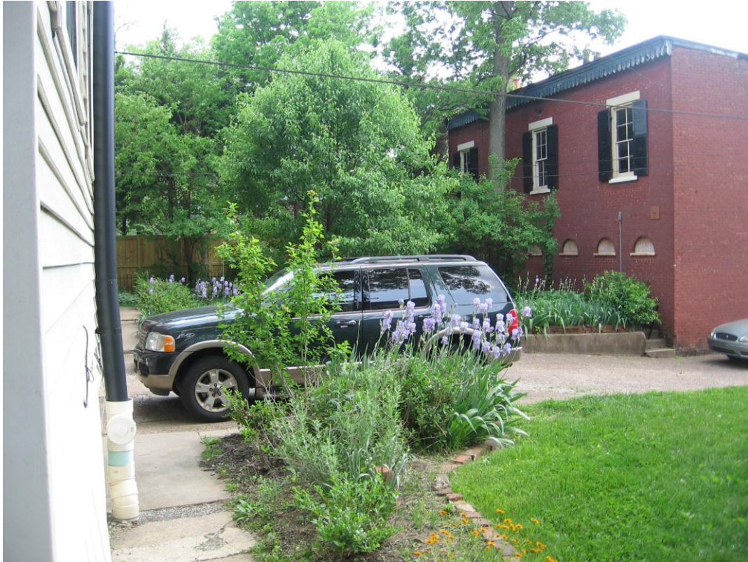
Carriage house at rear of property/ Private yard area and existing parking
