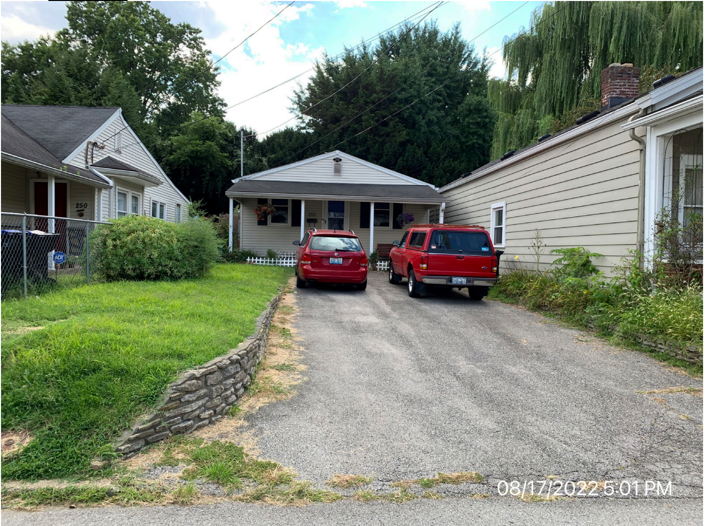
Front of subject property and off-street parking.
