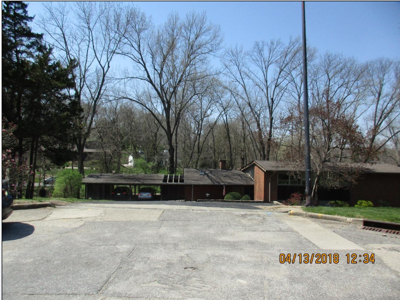
The front of the principal structure facing Brookside Drive.
