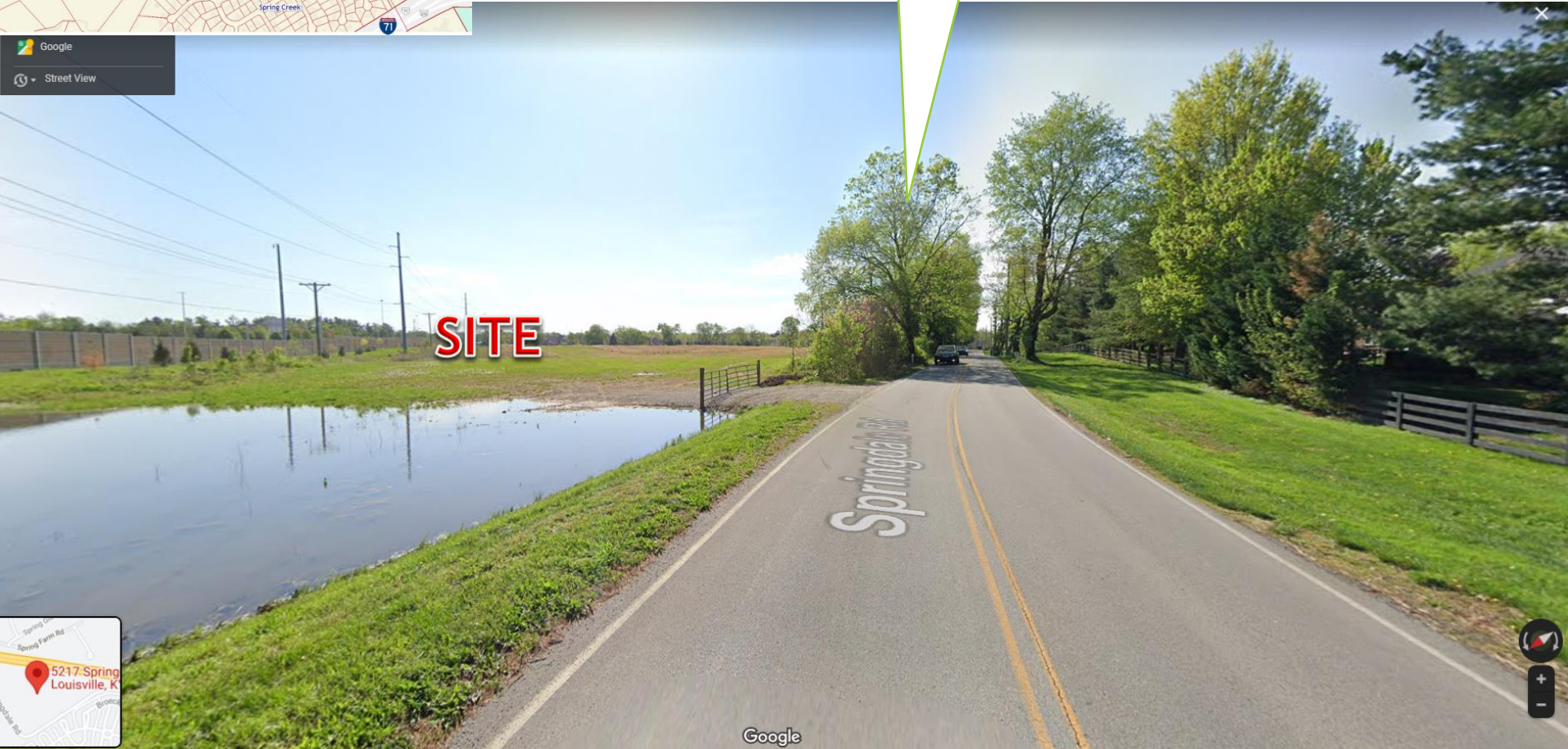
View of site from Springdale Road looking southeast.
