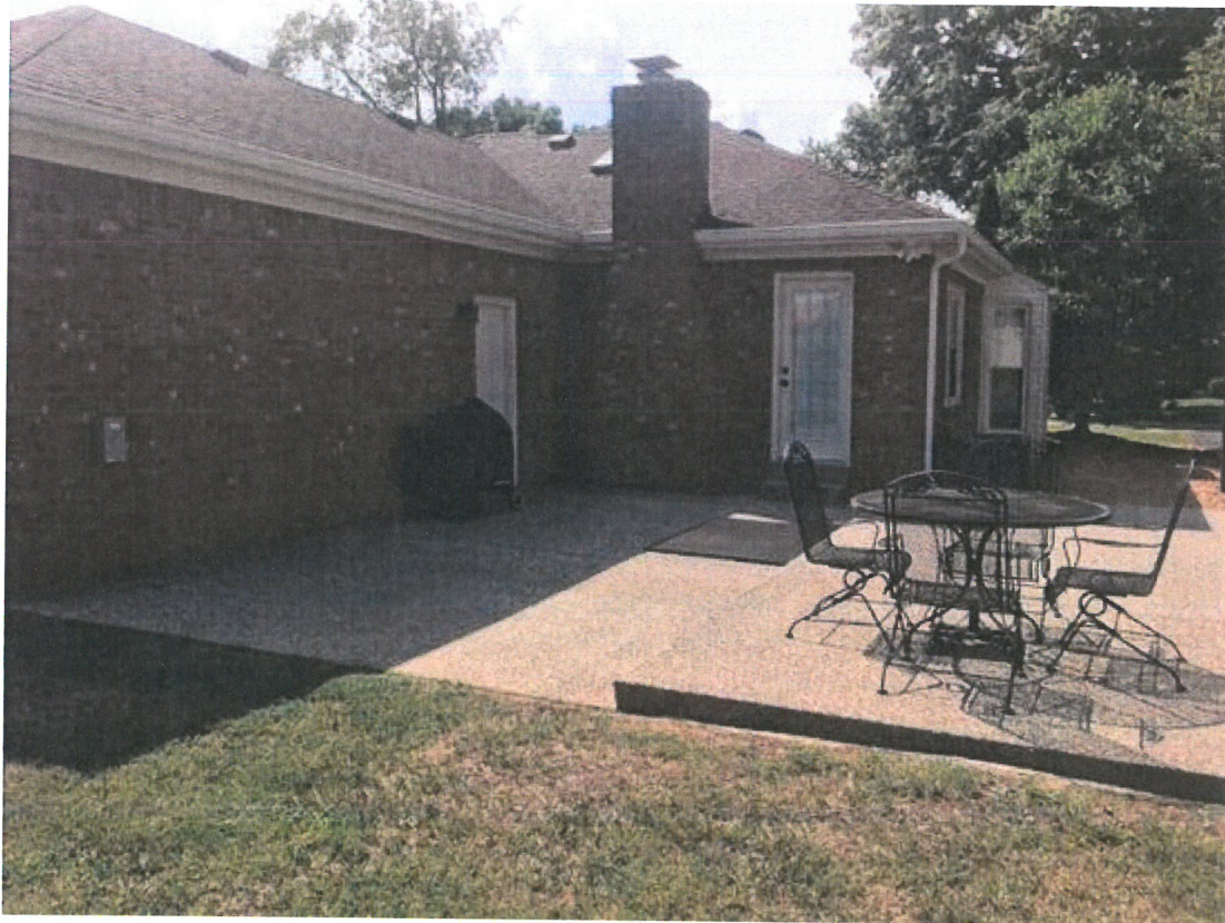
after the deck was built
