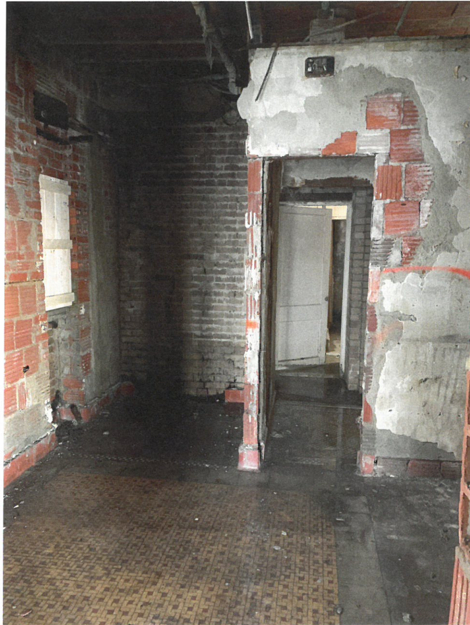
EXISTING BASEMENT DINING/KITCHEN
