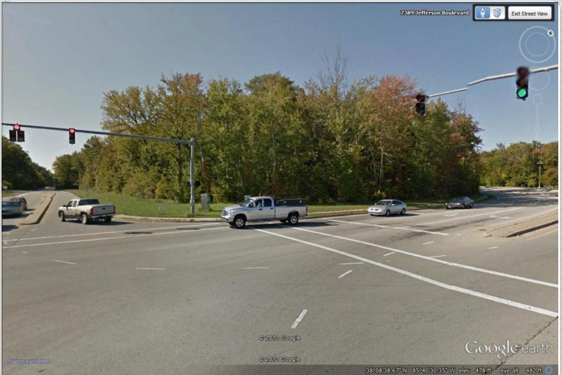
Intersection of McCawley Rd. and Jefferson Blvd.
